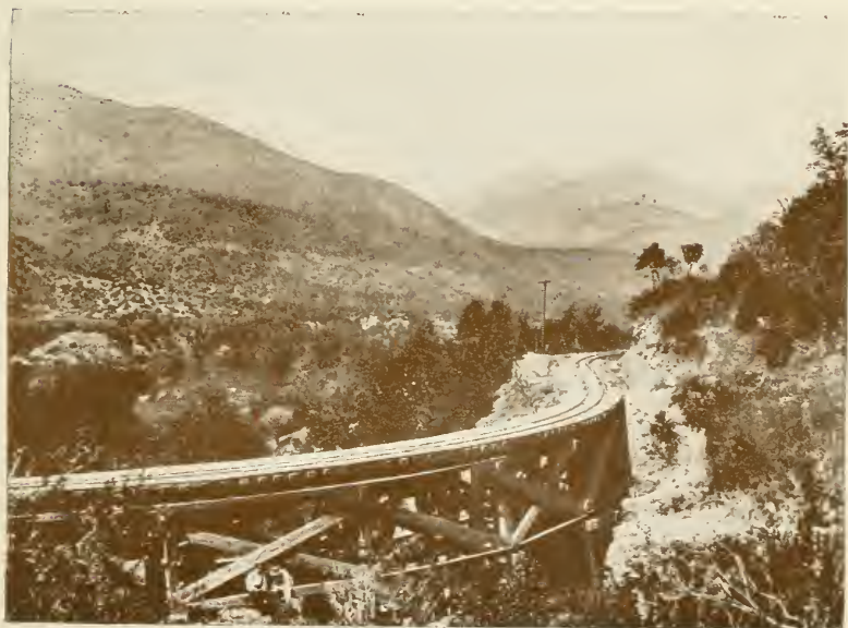
Railway between Rancagua and El Teniente.
