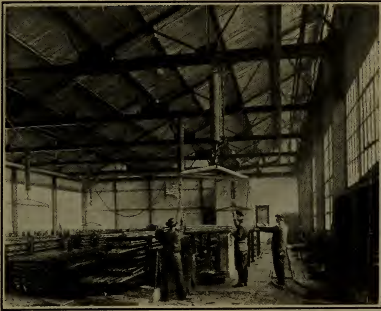
Fig. 248—Vertical cylinder hoists traveling on roof trusses employed in the warehouse of the Peerless Drawn Steel Co., Massillon, Ohio.
