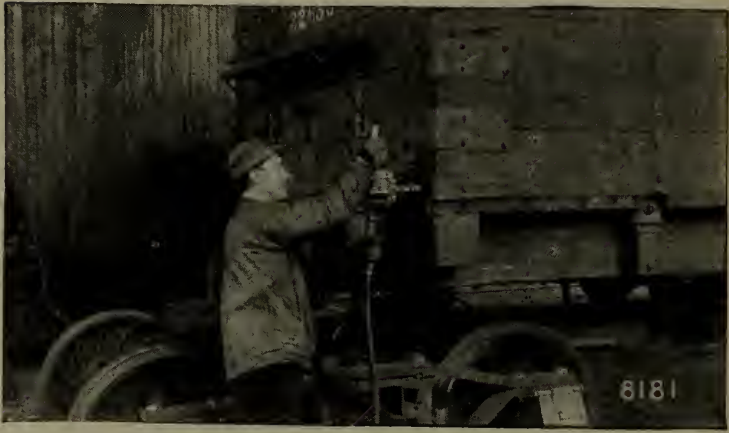
Fig. 195—Running up \frac{1}{2} -inch nuts on car corner straps with a pneumatic drill in the Collingwood-Ashtabula Shops, N. Y. Central R. R.
