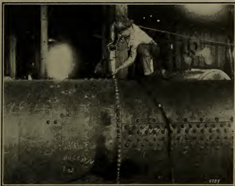
Fig. 204—Little David Riveter on boiler work in the Murphy Boiler Works, New Orleans, La.
