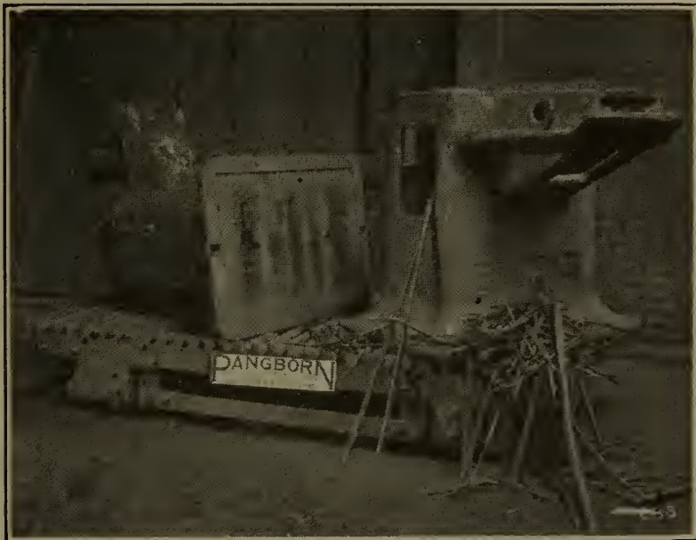
Fig. 134—Sand Blast Car.
