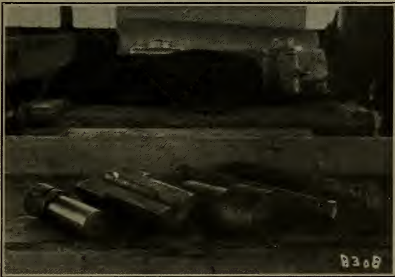
Fig. 185—Dies and dolly for forging bolt heads and sample of stock and finished work.
