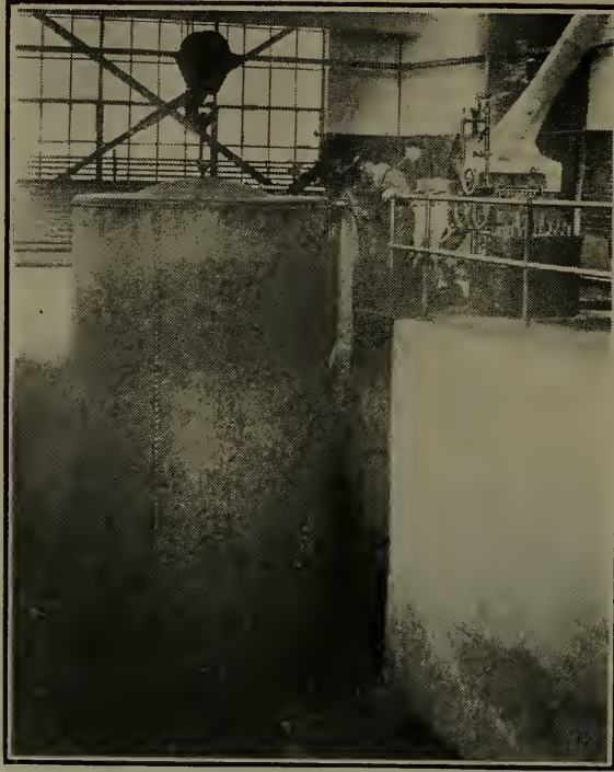
Fig. 217—A Hanna Pneumatic Yoke Riveter in the plant of the General Electric Co., Pittsfield, Mass., employed on transformer work.
