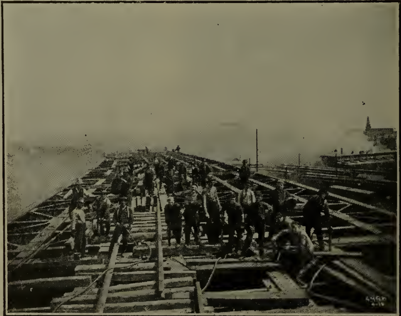
Fig. 212—Pneumatic riveters at work on a large railroad viaduct.
