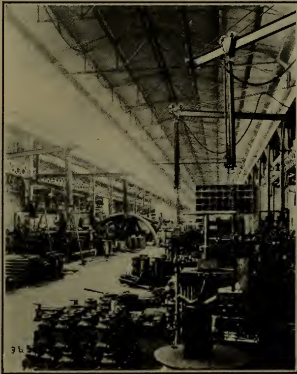
Fig. 242—Vertical cylinder hoists on swinging cranes serving machine tools.
