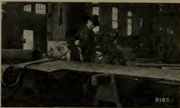
Fig. 205—Riveting angle iron on locomotive running board. Rivets \frac{3}{4} -inch diameter, driven cold with a medium weight chipping hammer.
