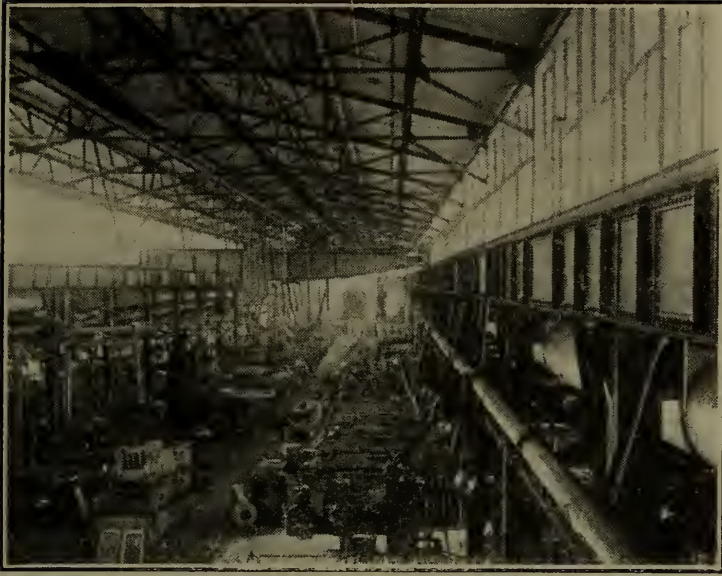
Fig. 234—A 20-ton pneumatic traveling crane in a large machine shop.
