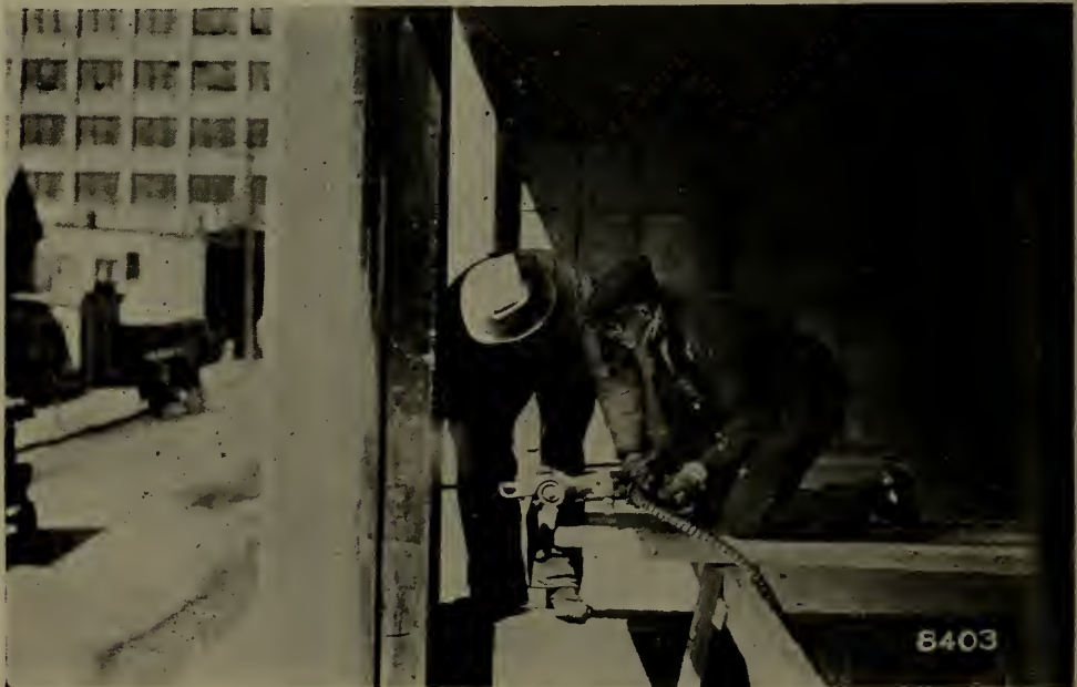
Fig. 86—Pneumatic hand rock drill for removing concrete and masonry foundations; drilling anchor bolt holes and digging trenches in rock formations. Illustration shows holes being drilled for window bolts in concrete, Edison Phonograph Co., Orange, N. J.
