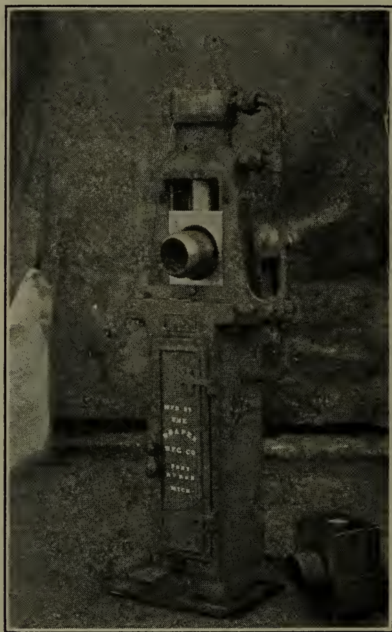
Fig. 226—Pneumatic boiler flue welding machine.
