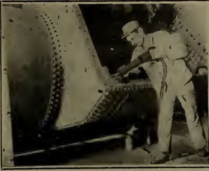
Fig. 223—Chipping mud-ring on locomotive boiler.
