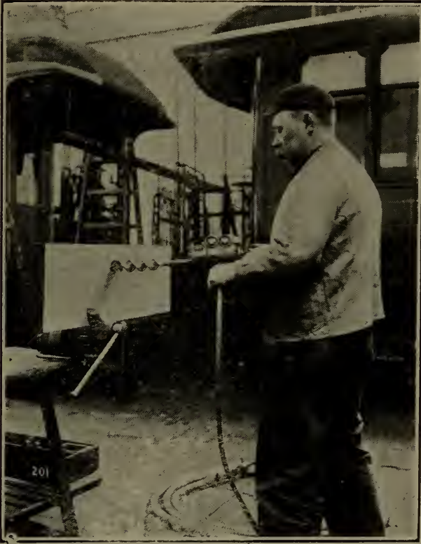
Fig. 199—Boring wooden end sills for passenger coaches.
