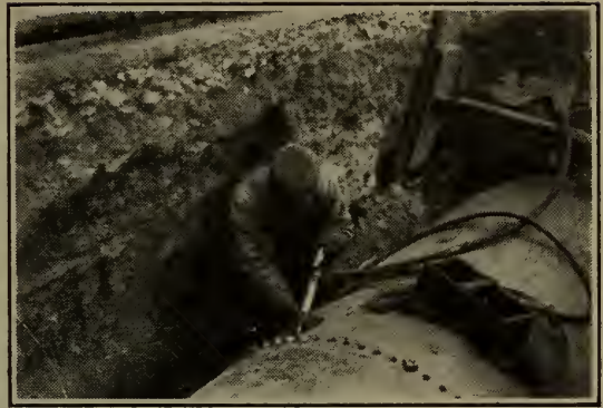
Fig. 224—Calking riveted steel pipe joints.
