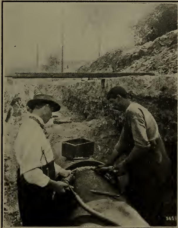
Fig. 225—Calking lead joints, cast-iron pipe line.
