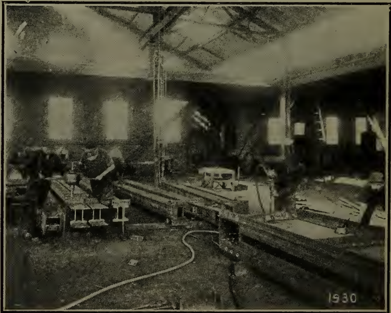
Fig. 202—Drilling and riveting structural steel shapes in a Brooklyn structural works.
