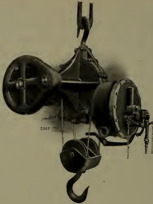
Fig. 54—Portable Geared Motor Hoist.
