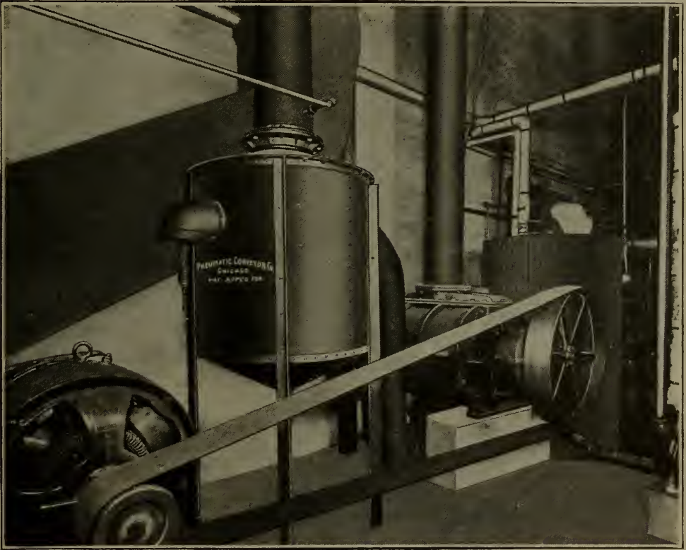
Fig. 250—Exhauster and air scrubber for pneumatic ash conveyer.
