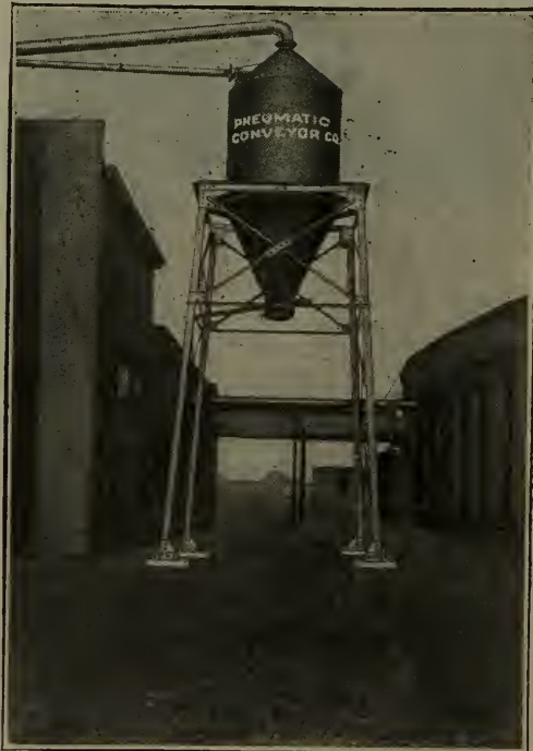
Fig. 252—Ash receiving tank.
