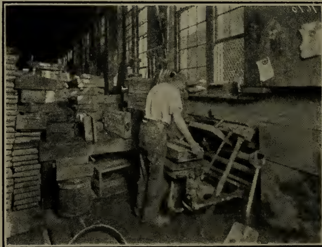
Fig. 101—Mumford power squeezing machine in the foundry of a New England Machine Tool Builder.
