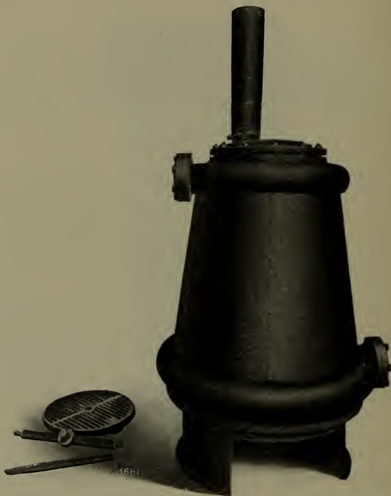
Fig. 47—A typical air reheater.
