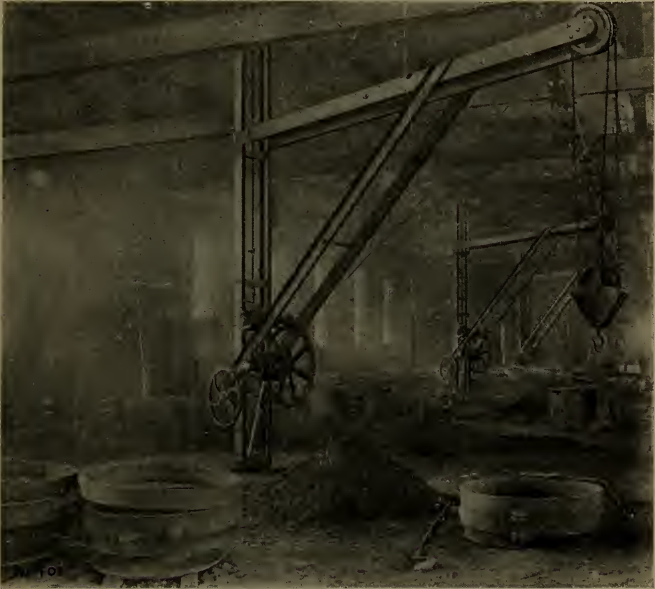
Fig. 239—Air powerized foundry crane, National Car Wheel Co., Sayre, Pa.
