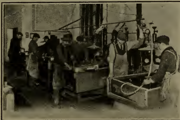
Fig. 228—Testing automobile radiators by air pressure in the plant of the Fedders Mfg. Co., Buffalo, N. Y.
