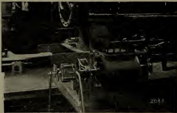
Fig. 162—Pneumatic drill employed with a special jig for re boring cylinders.
