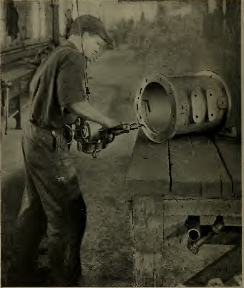
Fig. 158—Pneumatic drill applied to seating cylinder studs.
