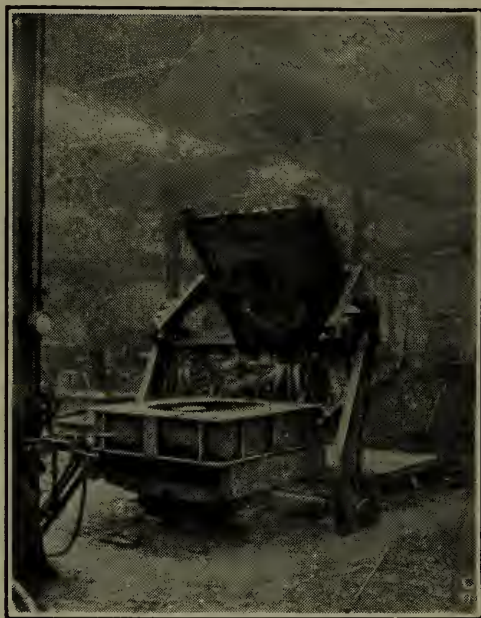
Fig. 107—Complete mold with pattern withdrawn.
