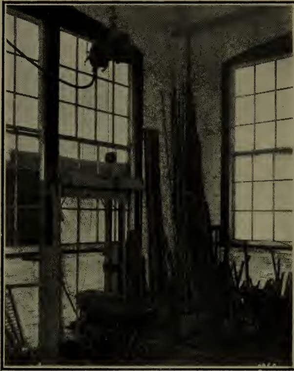
Fig. 240—Air motor hoist applied to elevator lift, City Forge & Iron Co., Dayton, Ohio.
