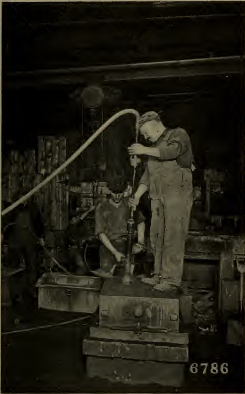
Fig. 91—Floor Sand Rammer used in conjunction with a pneumatic jarring machine.
