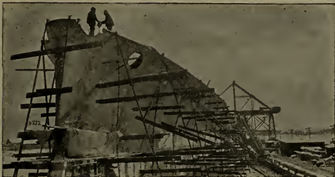
Fig. 193—A pneumatic drill at work drilling and reaming holes on a large battleship.
