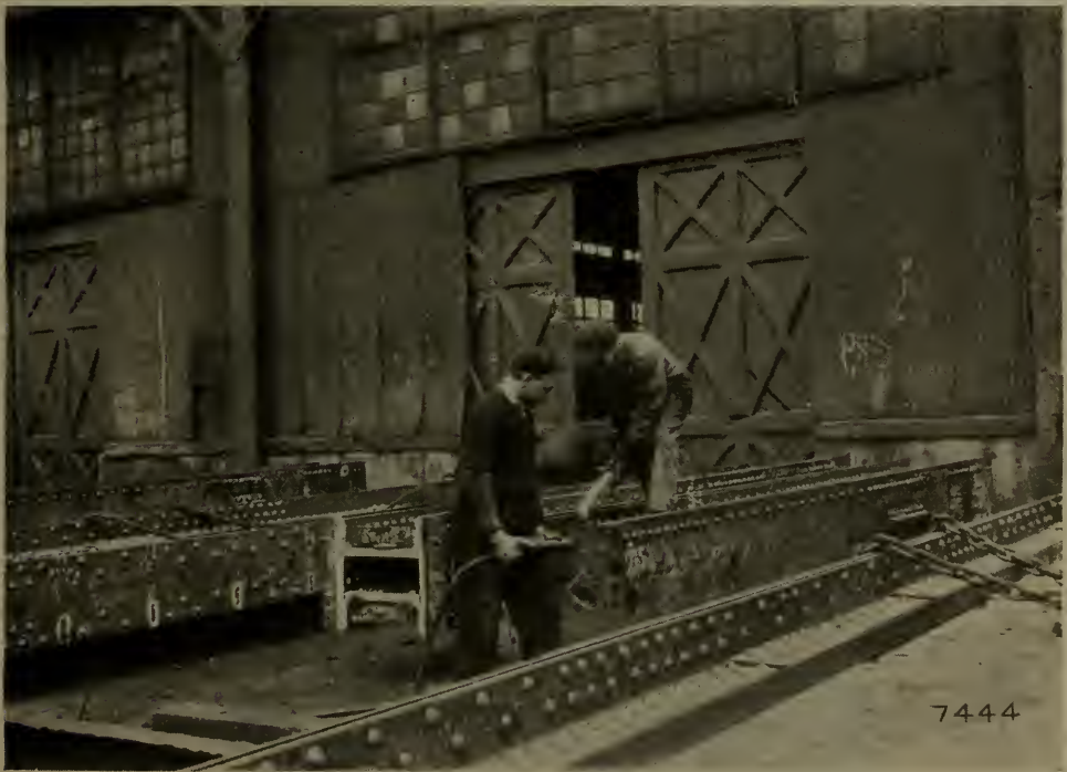
Fig. 220—Cutting off projecting ends of countersunk rivets on large structural columns. Hay Fdy. & Machine Wks., Newark, N. J.
