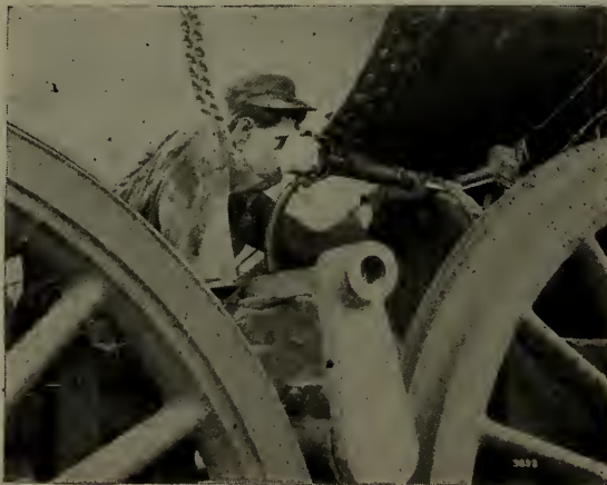
Fig. 222—Calking air drum underneath locomotive boiler.
