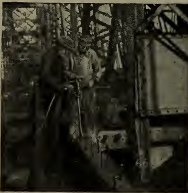
Fig. 198—Tightening bolts in guard rail on Louisville Bridge.
