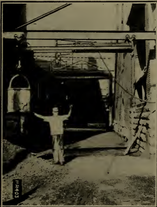
Fig. 88—Removing ashes from pit underneath boiler by means of a pneumatic horizontal cylinder hoist, operating from an overhead trolley runway.
