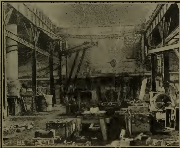
Fig. 235—Pneumatic traveling crane and powerized stationary crane in a foundry.
