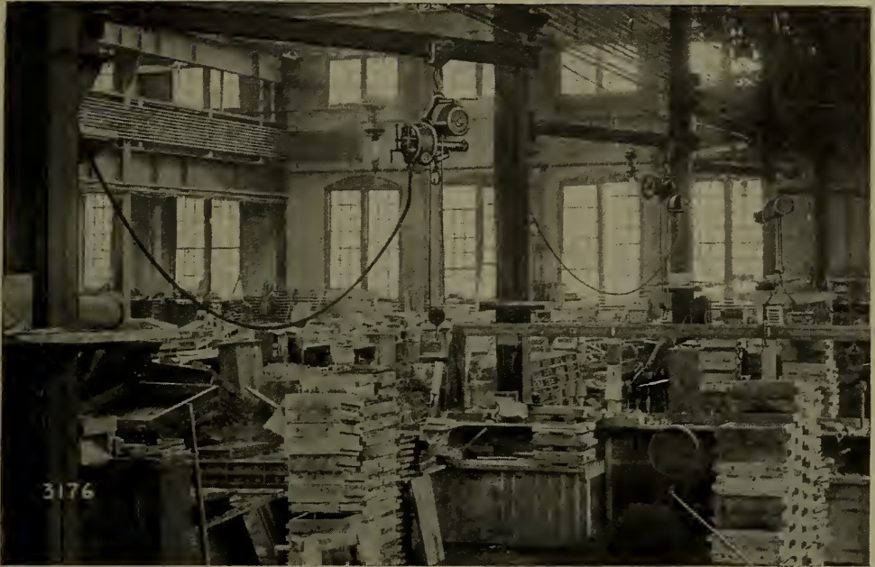
Fig. 118—View in the foundry of the Pratt & Whitney Co., Hartford, Conn. Both motor and cylinder hoists are used in conjunction with swinging post cranes as auxiliaries to a large traveling crane.
