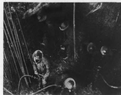
SULLIVAN ROTATOR HAMMER DRILLS 1,700 FT. UNDERGROUND, SINKING THE OTTAWA SHAFT OF THE MONTREAL MINING CO. HURLEY, WIS.
