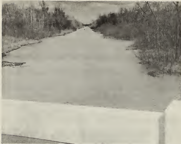
East side of bridge over Loosahatchie River on the Raleigh-Millington Road. Note straight, even flow without obstructions.
