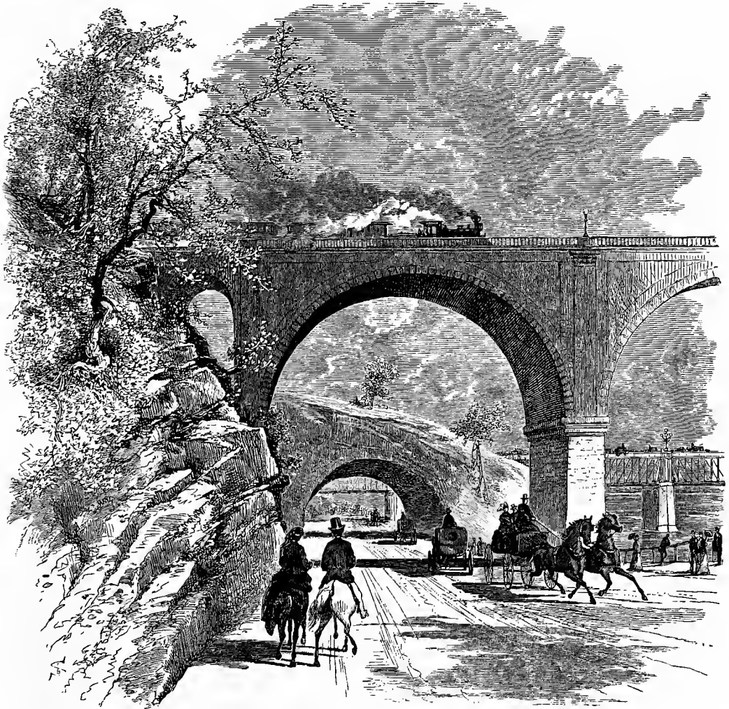
BRIDGE AND TUNNEL IN FAIRMOUNT PARK.
