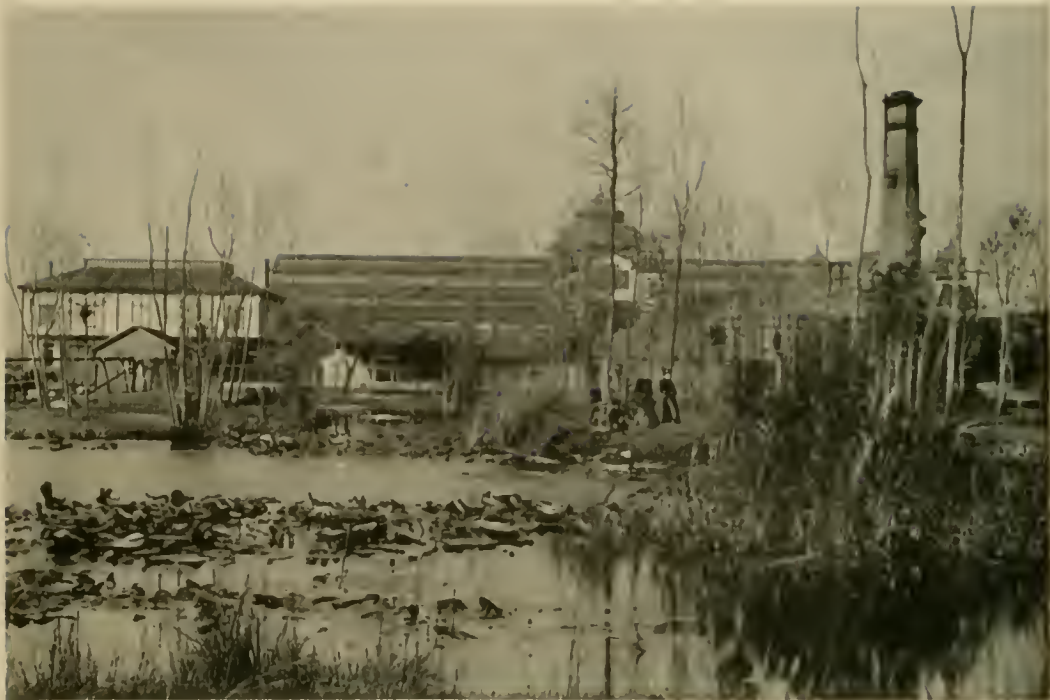
VIEW AT THE WATER WORKS.
