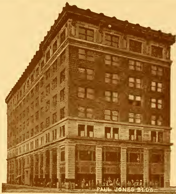
THE PAUL JONES BLDG., FOURTH AND JEFFERSON.
