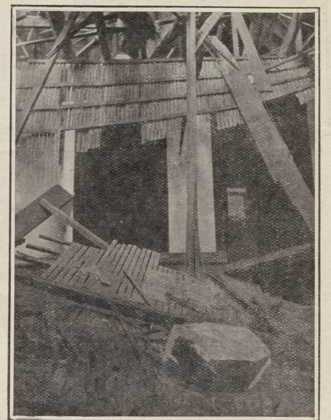
EFFECTS OF THE EARTHQUAKE. Another interior view at the Seminary.
