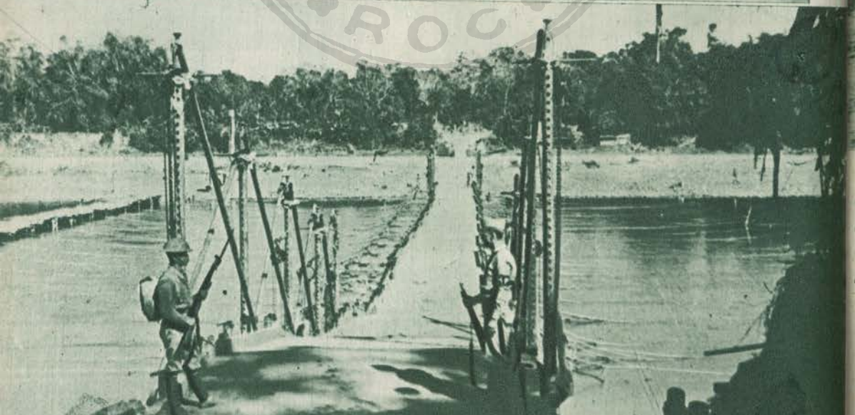
于前次戰事攻下以後，大龍河上的橡皮橋 迅速架設起來，由國軍及美憲兵共同護守。 Chinese soldiers together with U. S. MPs guard- ing a pontoon bridge erected on Tarun Hka after the capture of Yupong Ga and Taibpa Ga.
