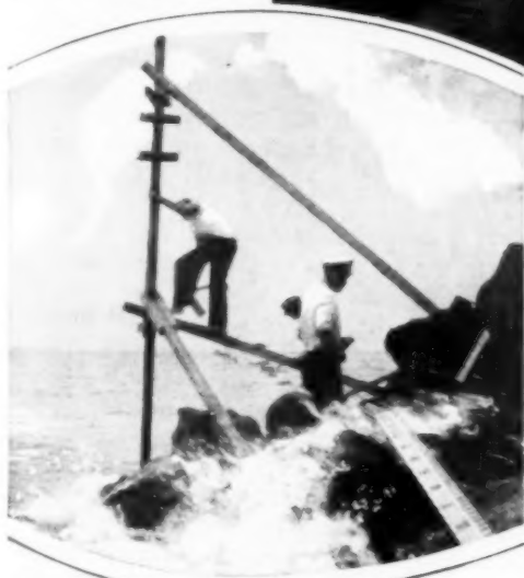
Courtesy U. S. Coast and Geodetic Survey Box Tide Gauge at Lynnhaven, Va.; Dr. Ralph E. Wilson, of the Carnegie Institution, with Device Illustrating Tides, and Workmen Erecting Gauge
