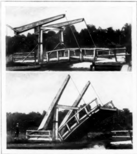
Old-Style Balanced Bridge Still in Use over a Canal within Twenty Miles of London, England
