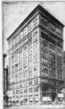
Our Pittsburgh Office Suite 514 Empire Building
