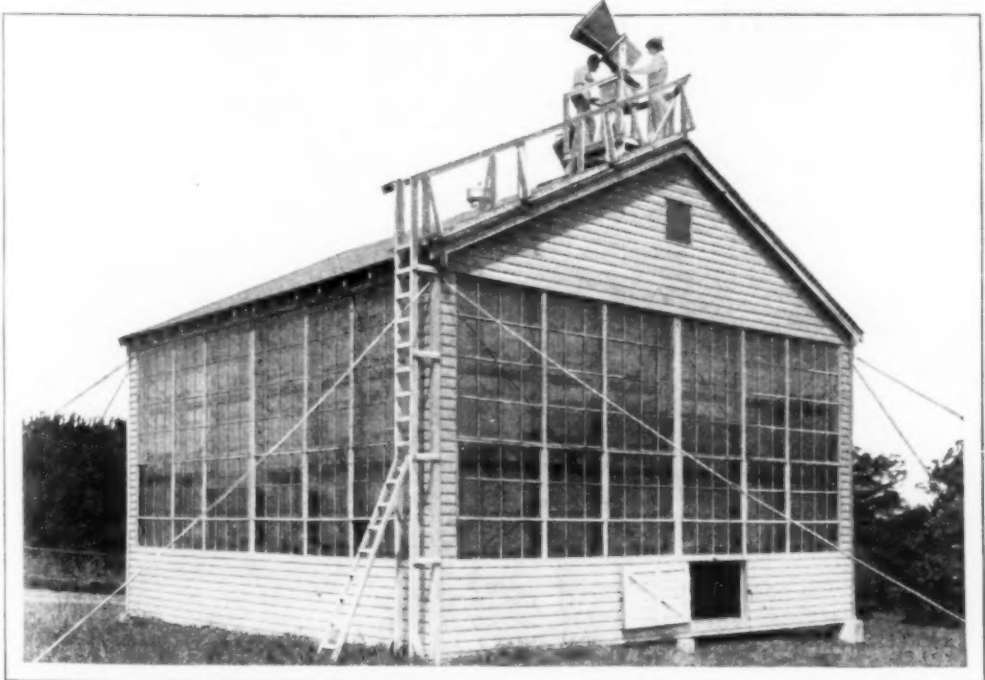
The Glass House in Which Uncle Sam Is Attempting to Solve the Problem of the Best Arrangement for Daylight Illumination; the Sunlight Recorder Is Shown on the Roof
