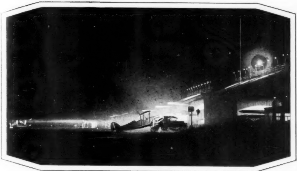
Night Lights On at the Oakland Airport; the Searchlight on Top of the Hangar Casts an 8,000,000-Candlepower Beam into the Air, While the Ground Light Is of 30,000,000 Candlepower
