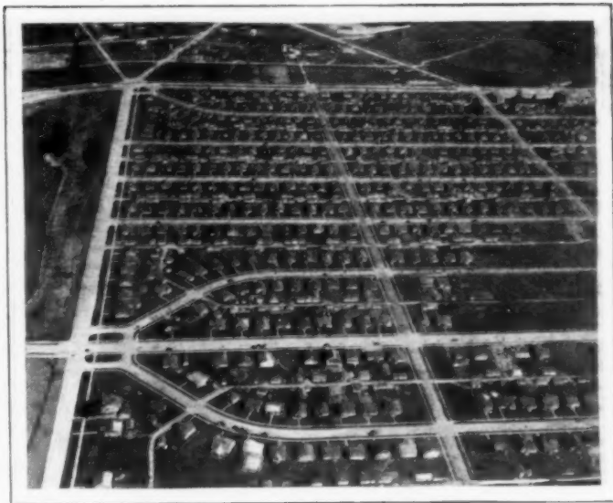
Model City Being Developed by Coast Lumber Company Has Unusual Street Layout for Its Garden Homes
