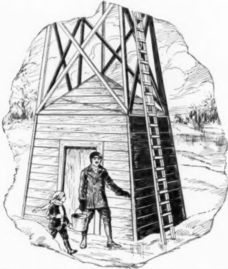
Wooden Inclosure Lined with a 12-In. Straw Wall Prevents Pump from Freezing
