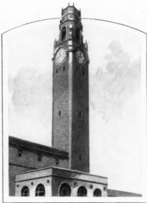
This Stately Clock Tower, Built as a War Memorial, Is Really the Chimney of a Heating Plant
