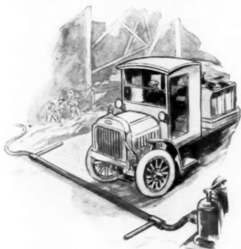
Length of Pipe Makes a Good Protector for Hose Laid over Busy Street
