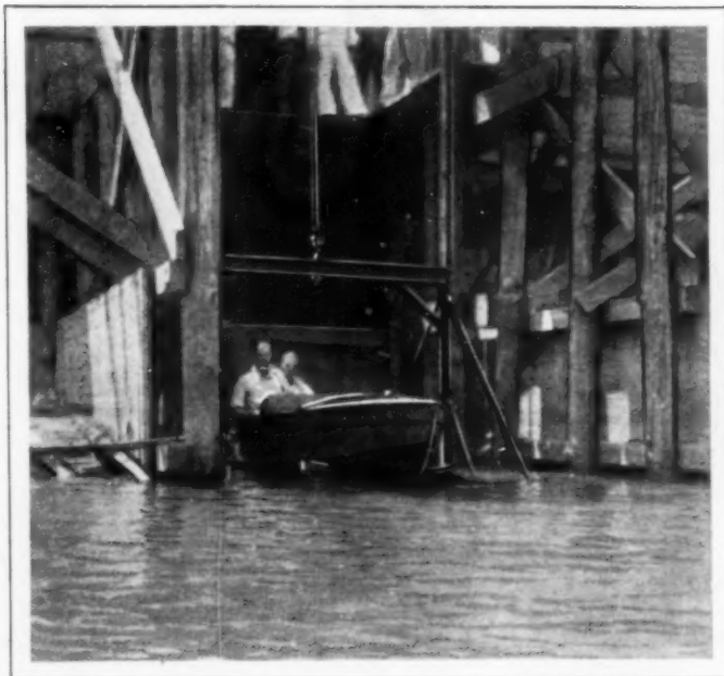
Electric Hoist for Elevating Boats from Illinois River to Docking Space on Bank; It Will Lift Two Tons
