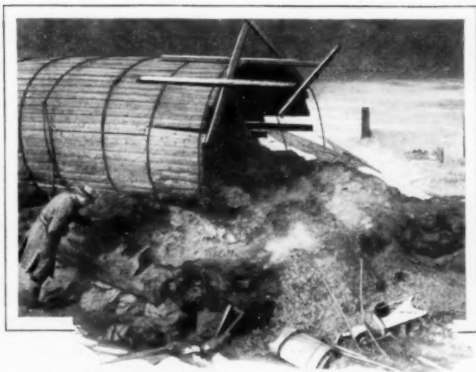
A Farm Silo near Middlesex, Vermont, Blown to Pieces as a Result of Spontaneous Combustion Igniting the Gases during Fermentation
