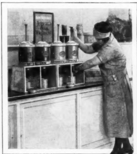
Food Dispenser Which Keeps Bulk Semiliquids in Sanitary Containers Instead of Open Jars
