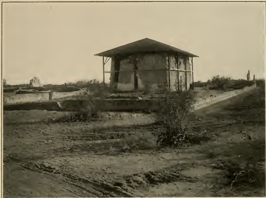
a View of west wall from northwest
