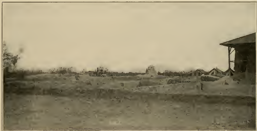
c View from outside north wall NORTHEAST BUILDING
