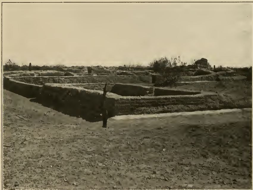
b View of northwest room from northwest
