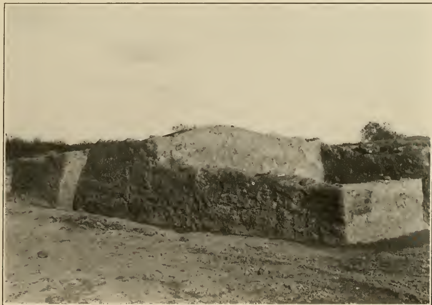
b View from northwest NORTHEAST BUILDING
