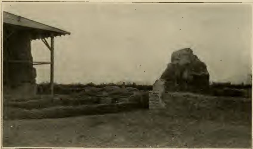
b View from same point after excavation
