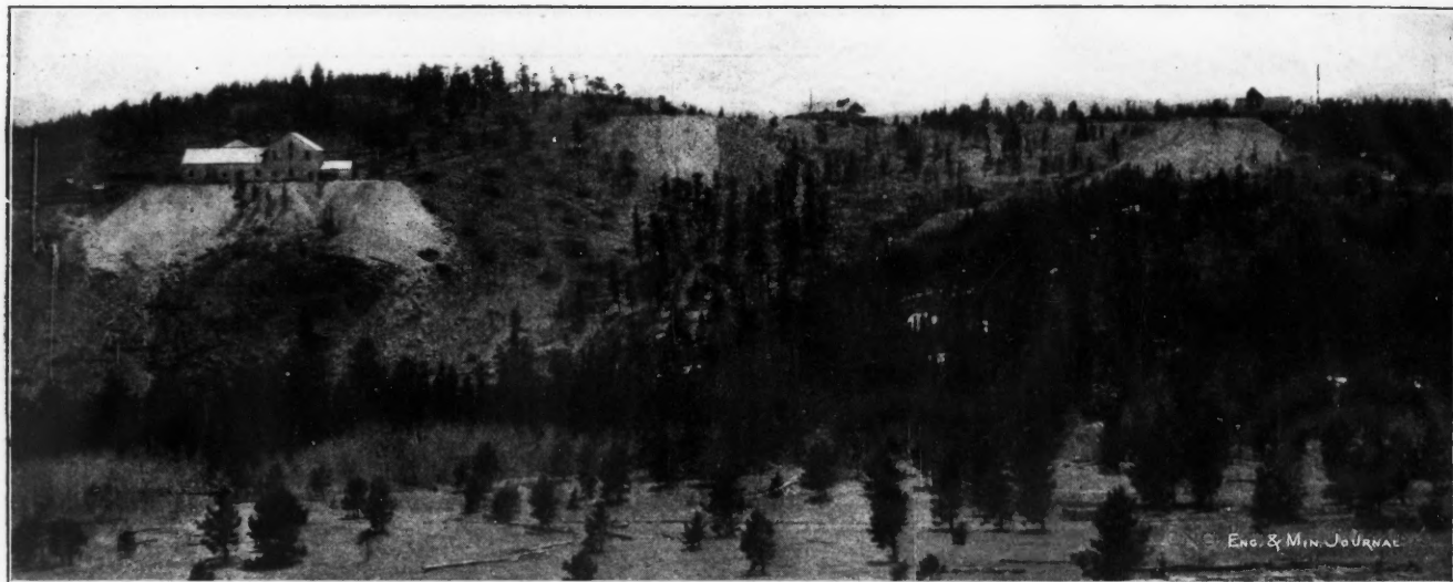
FIG. 6. CONGER SHAFT HOUSES
