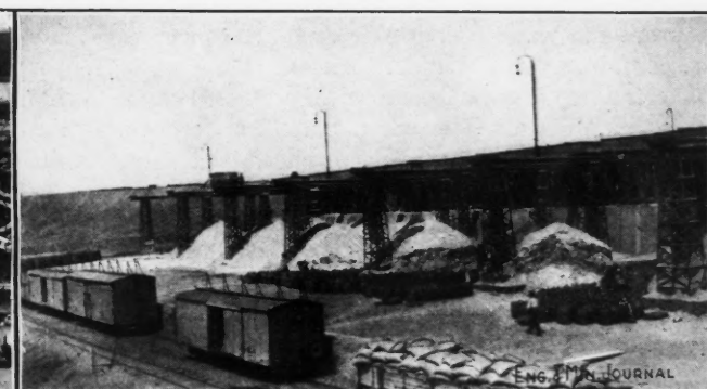
NITRATE READY FOR BAGGING AND SHIPMENT Nitrate is brought from bateas in steel cars.
