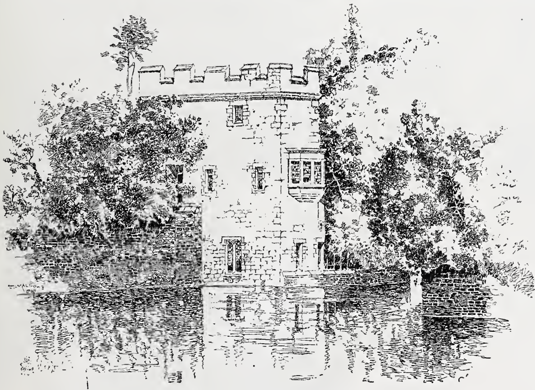
GATE-HOUSE AND MOAT TO THE BISHOP'S PALACE, WELLS.
