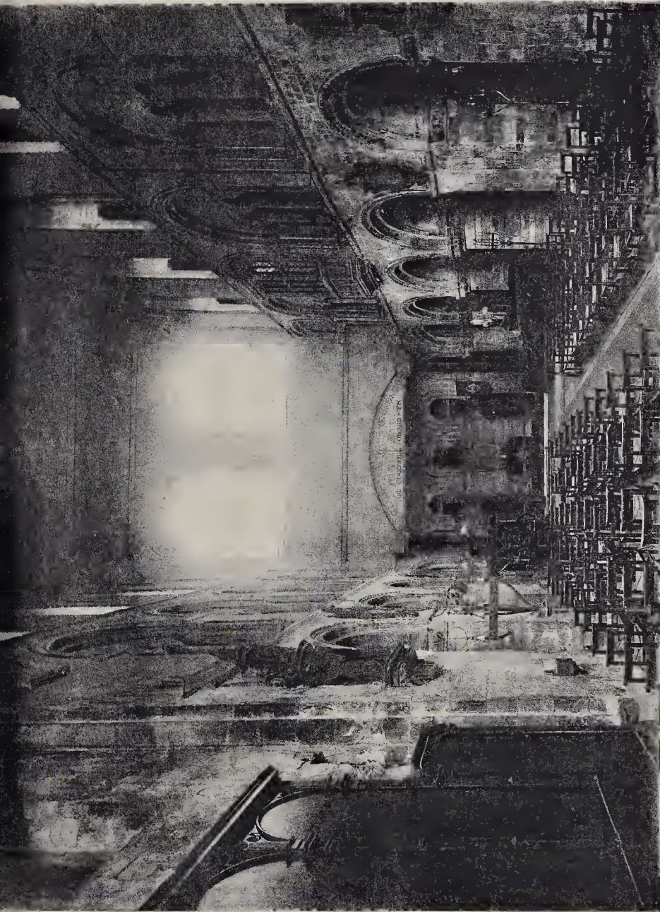
ST. BARTHOLOMEW THE GREAT, SMITHFIELD INTERIOR LOOKING EAST, SHewing IRON COLUMNS FOR SUPPORTING FACTORY BUILDING EXTENDING OVER THE AISLE.
