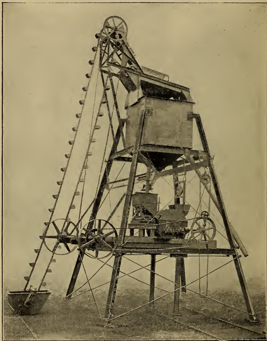
FIG. 22.— Semi-portable Mixing Platform.
