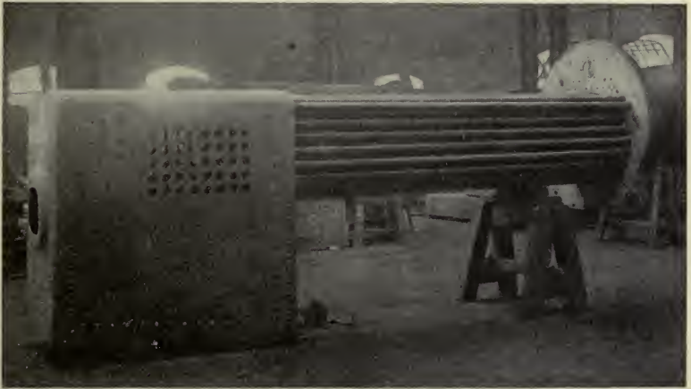
BOILER IN COURSE OF CONSTRUCTION
