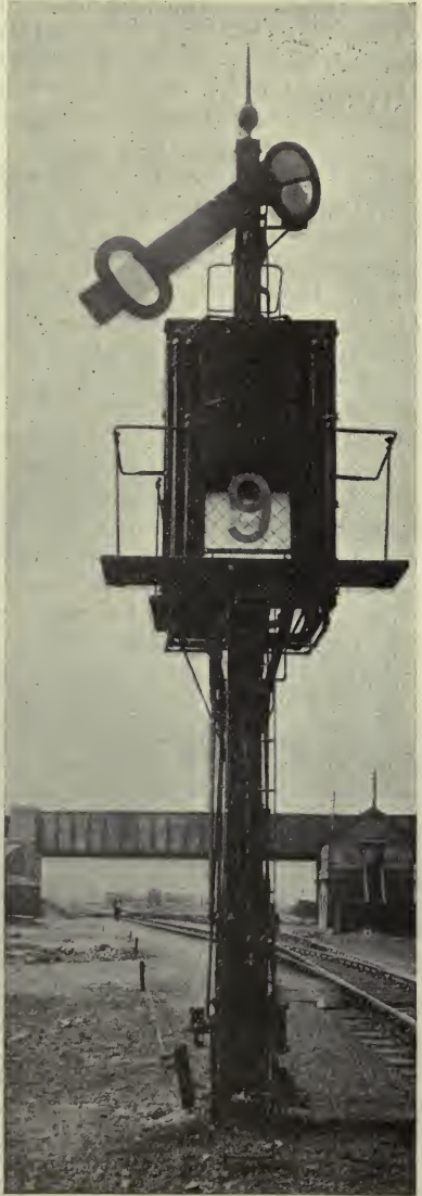
GOODS AUTOMATIC SIGNAL Controlling ten roads (Wath Concentration Sidings, G.C.R.)
