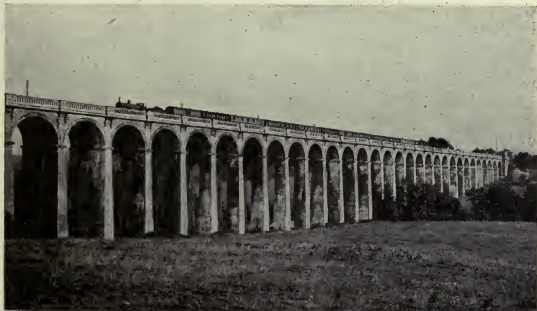
OUSE VALLEY VIADUCT (London, Brighton, and South Coast Railway)
