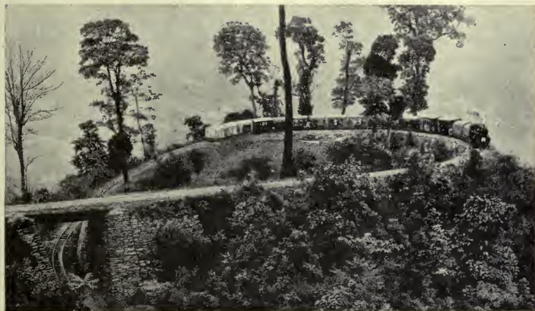
A TRAIN TRAVERSING A MOUNTAIN "LOOP" (Darjeeling Railway)
