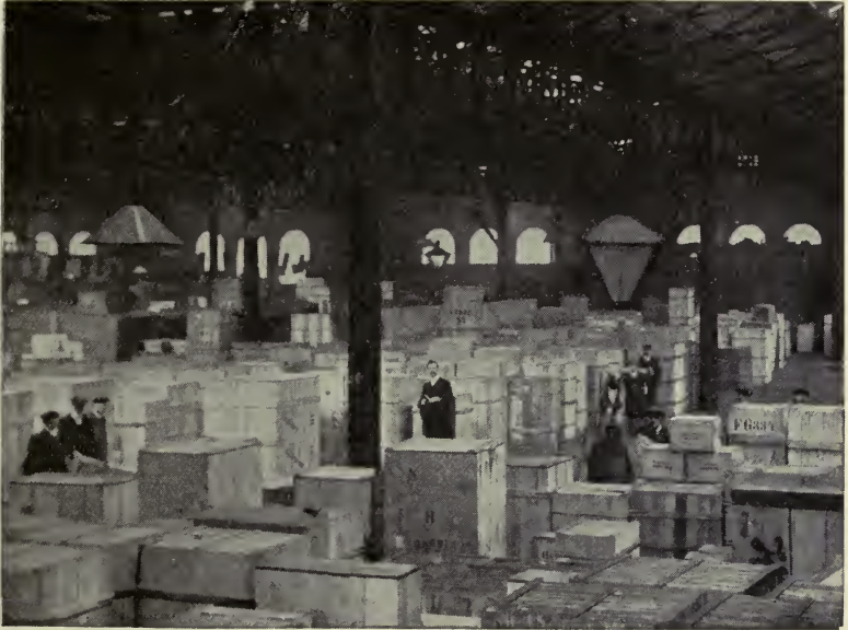
PORTION OF CONTINENTAL WAREHOUSE, BISHOPSGATE GOODS STATION (Great Eastern Railway)
