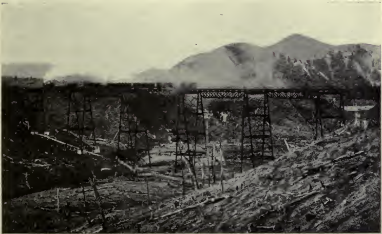
MANGAWEKA VIADUCT (New Zealand Government Railways)
