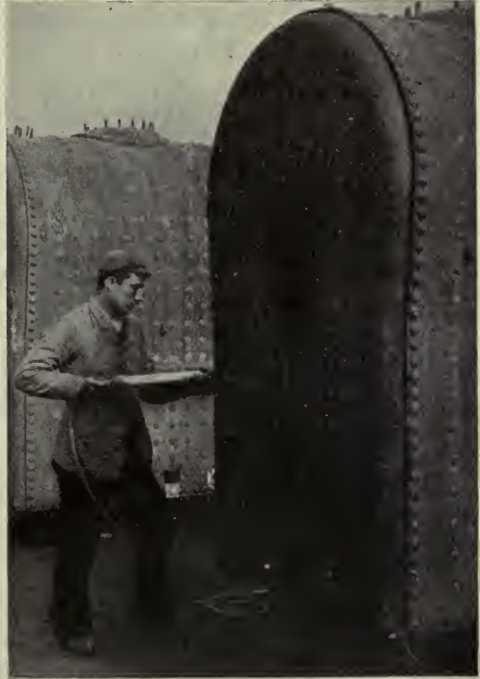
PNEUMATIC RIVETING AT STRATFORD WORKS (Great Eastern Railway)
