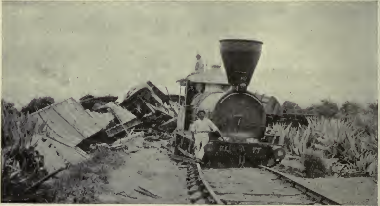
AN ACCIDENT CAUSED BY THE SUBSIDENCE OF THE LINE AFTER A FLOOD ON AN INDIAN RAILWAY
