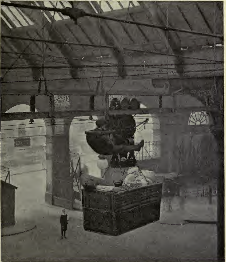
OVERHEAD TRANSIT AT VICTORIA STATION, MANCHESTER (Lancashire and Yorkshire Railway)
