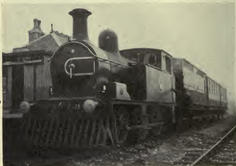
0-6-0 TANK ENGINE FITTED WITH "COW CATCHER" (Great North of Scotland Railway)
