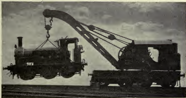
BREAK-DOWN CRANE-ENGINE LIFTING A LOCOMOTIVE (North Eastern Railway)
