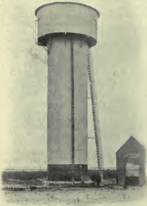
WATER-SOFTENER AT ALDERMASTON (Great Western Railway)
