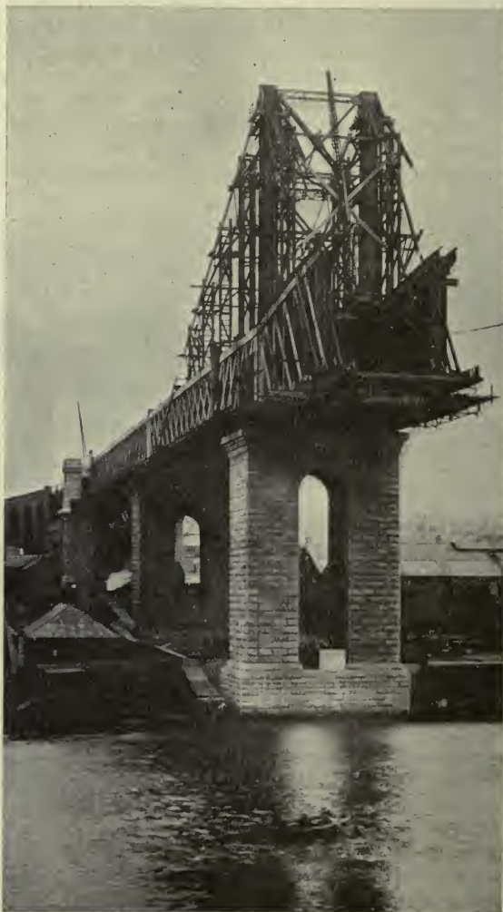
QUEEN ALEXANDRA BRIDGE, SUNDERLAND Cantilever in course of erection
