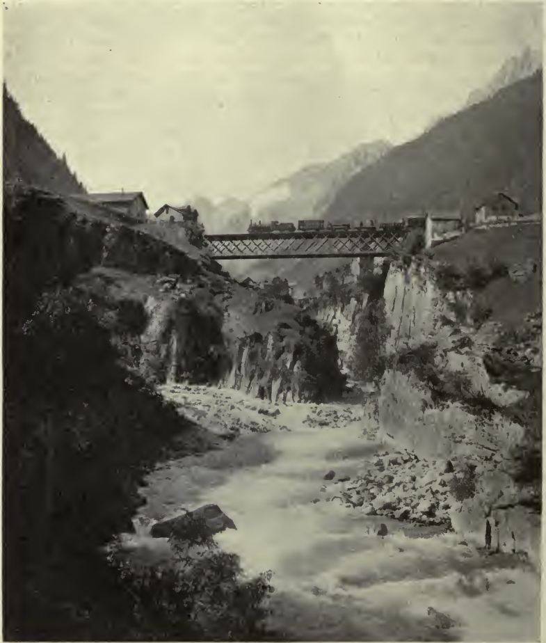
GOSCHENEN VIADUCT, GOTHARD RAILWAY (Swiss Federal Railways)
