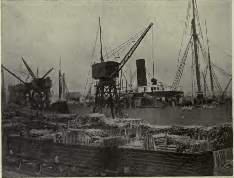
ELECTRIC CRANES DISCHARGING TIMBER (PIT PROPS) AT HARTLEPOOL (North Eastern Railway)
