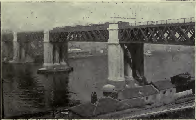
A TRAIN OF 14 ENGINES AND 12 TENDERS Testing King Edward's Bridge, September 29th, 1906 (North Eastern Railway)
