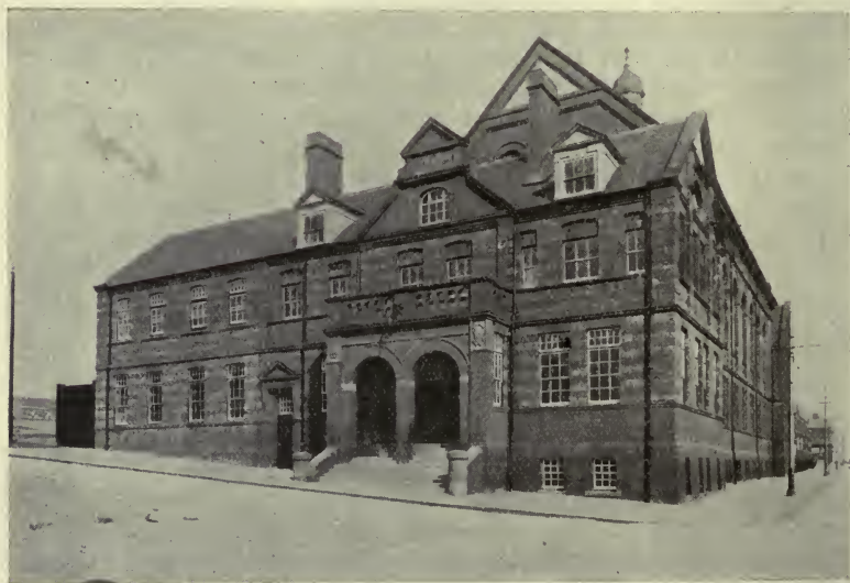
MECHANICS' INSTITUTE, HORWICH (Lancashire and Yorkshire Railway)
