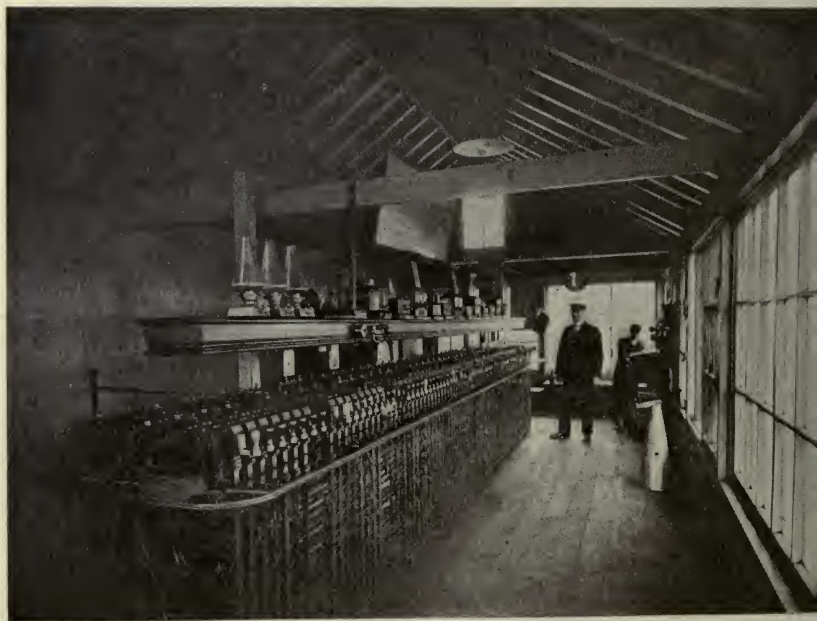
SIGNAL-BOX ENTRANCE TO WATERLOO (L.S.W.R.) PNEUMATIC SIGNALLING APPARATUS, LONDON ROAD, MANCHESTER (G.C.R.)
