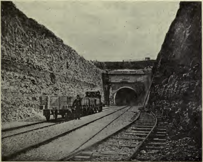
SEVERN TUNNEL, ENTRANCE ON WELSH SIDE
