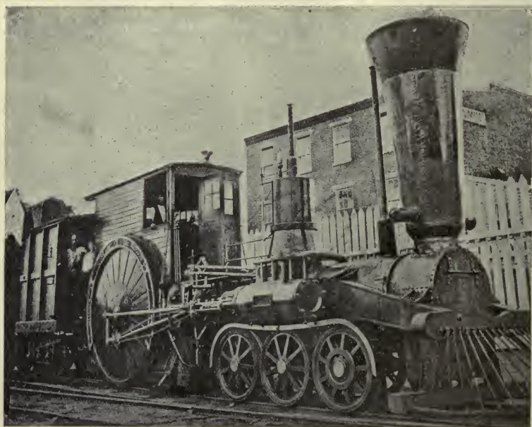
AN OLD EIGHT-FOOTER (Camden and Amboy Road, 1845)
