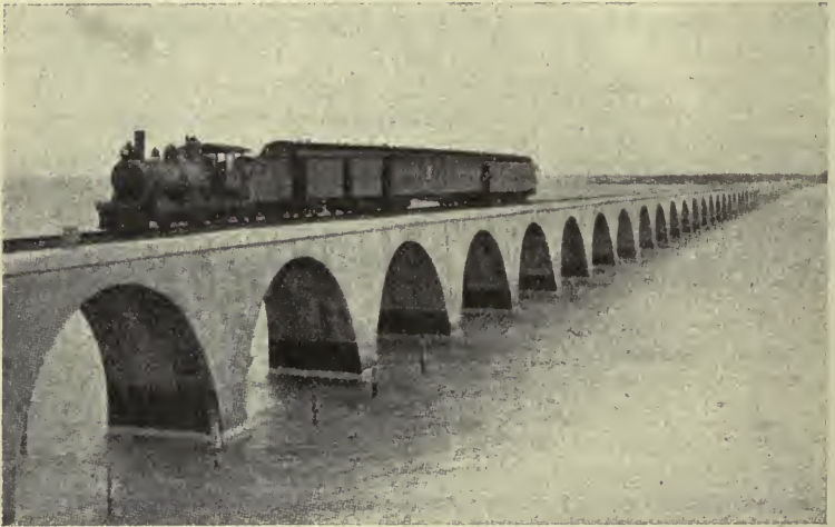
VIADUCT ACROSS AN ARM OF THE ATLANTIC OCEAN (Florida East Coast Railroad)
