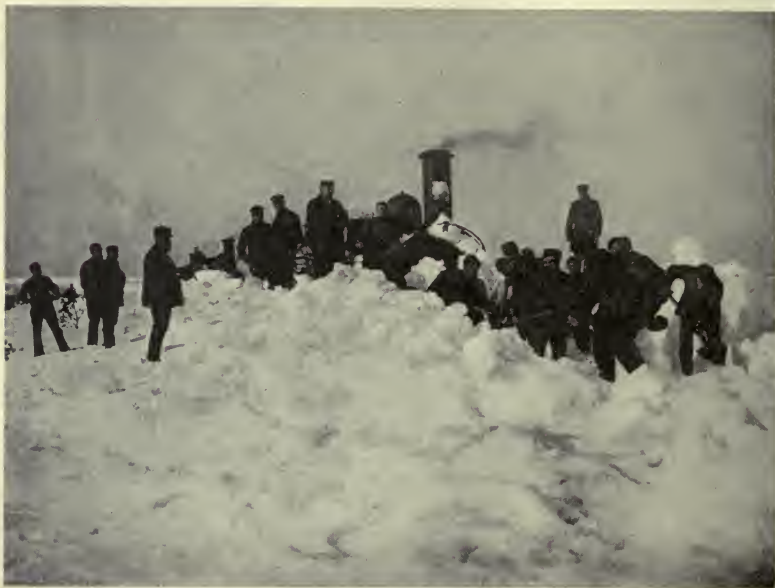
SNOW PLOUGH BLOCKED IN A DRIFT (Highland Railway)
