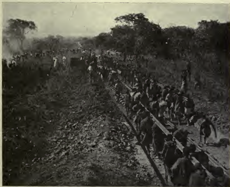
RAILWAY CONSTRUCTION IN RHODESIA
