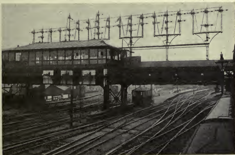
SIGNAL GANTRY, ENTRANCE TO WATERLOO STATION (London and South Western Railway)
