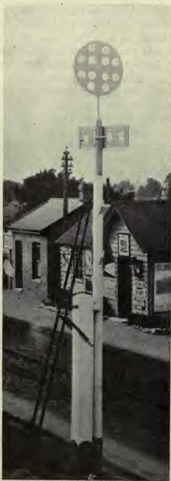
OLD DISC SIGNAL Recently standing at Spetisbury (Somerset and Dorset Joint Railway)
