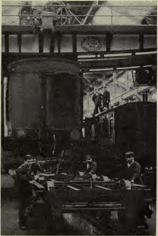
CARRIAGE-LIFTING, WOLVERTON WORKS (London and North Western Railway)
