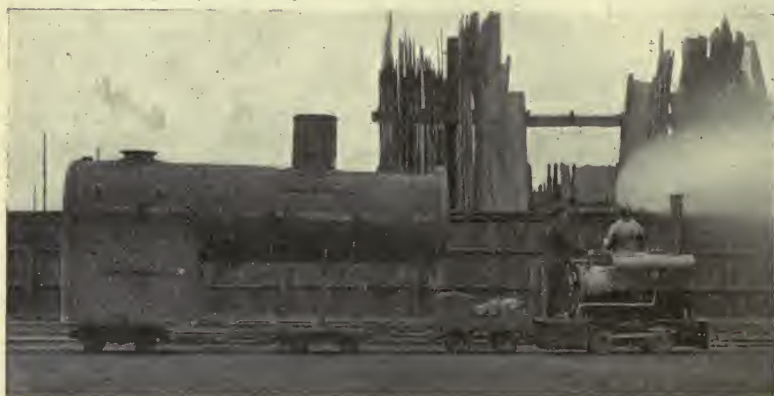
A TRAMWAY LOCOMOTIVE For hauling materials at Horwich Locomotive Works (Lancashire and Yorkshire Railway)
