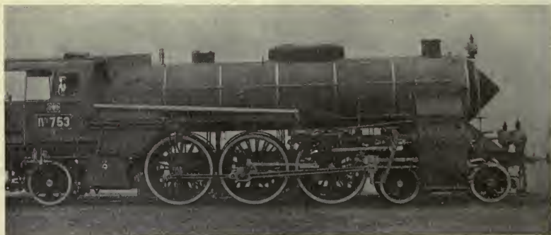
4-6-2 FOUR-CYLINDER COMPOUND LOCOMOTIVE (Bavarian State Railways)
