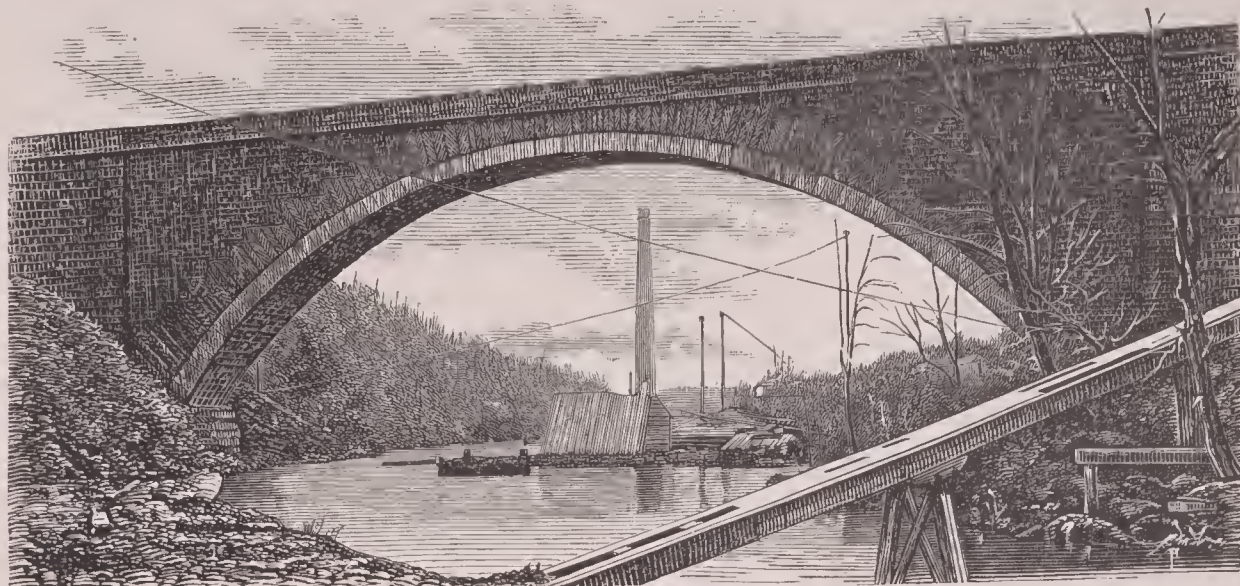
Cabin John arch.
