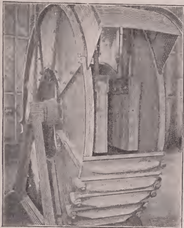
Front of Horry furnace.
