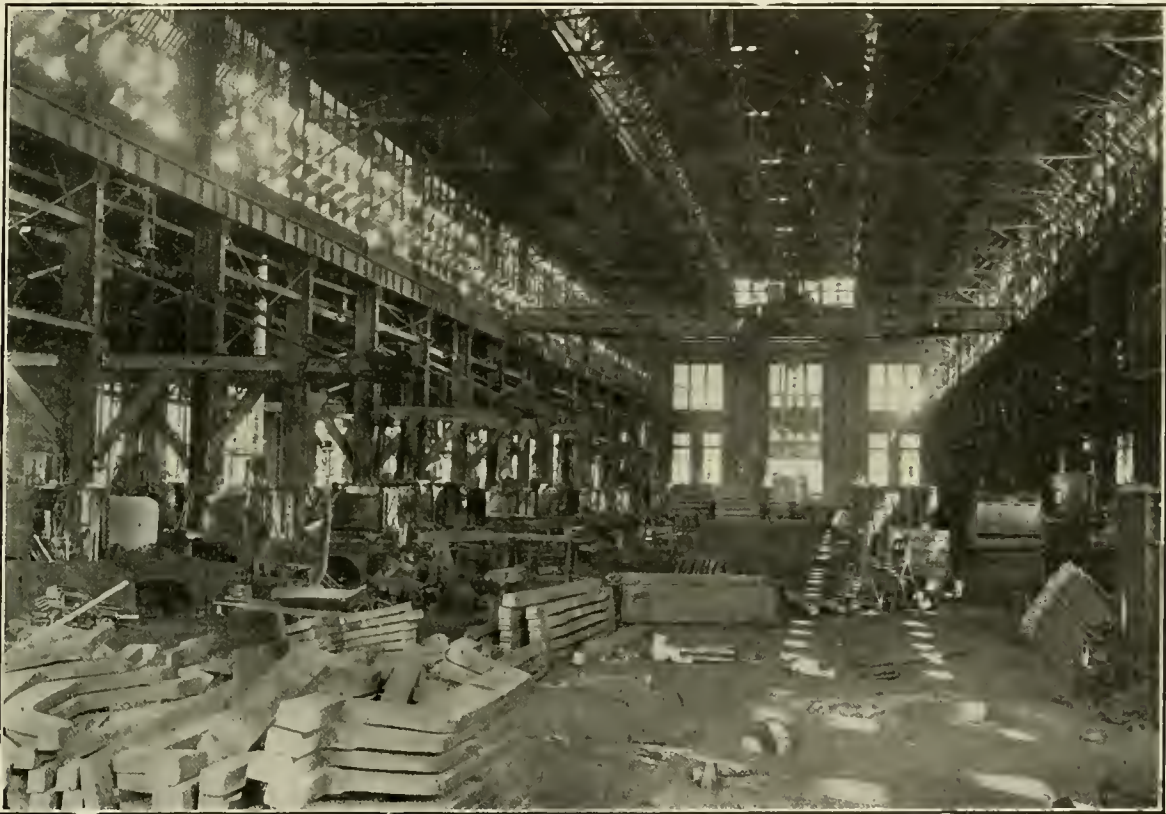
CENTRAL BAY OF SMITH SHOP.—SOUTH LOUISVILLE SHOPS.
