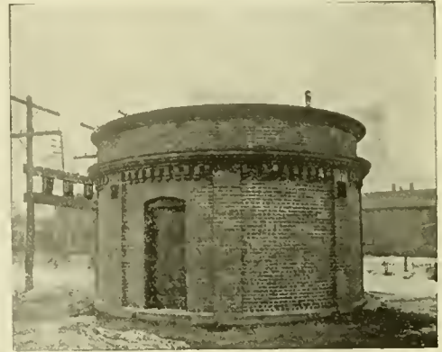
FIG. 1—ELECTRIC PUMPING STATION.
