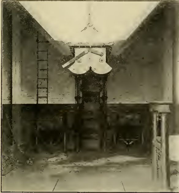
BOTTOM OF COAL SUPPLY BIN.
