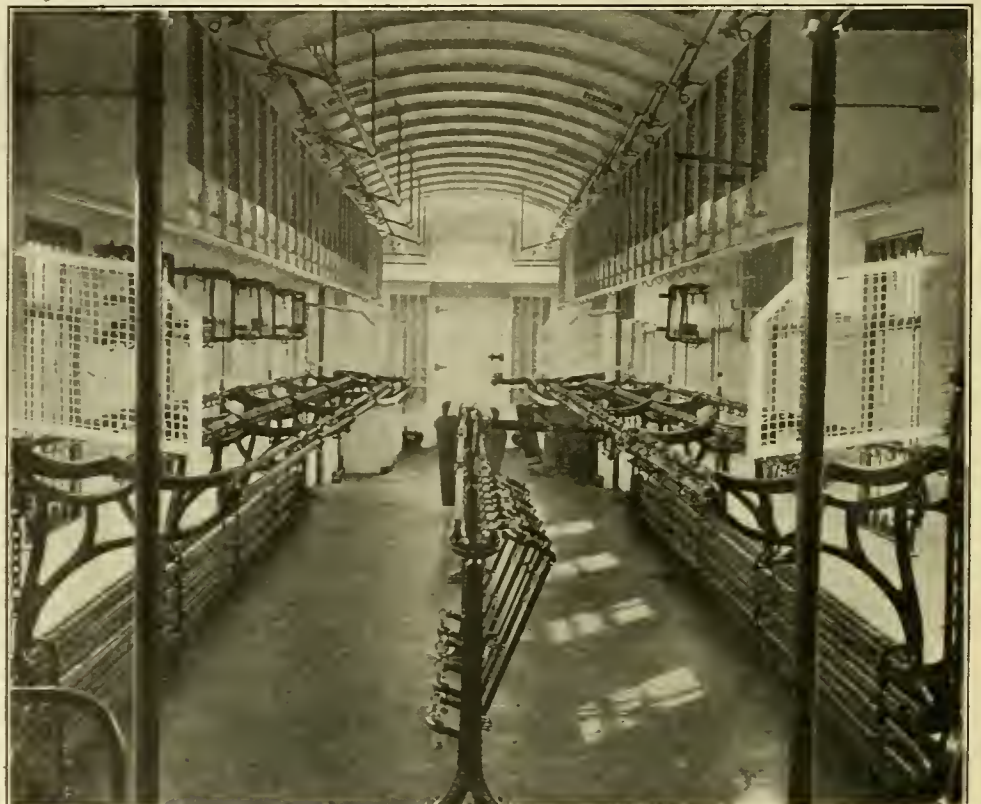
INTERIOR OF ALL-STEEL POSTAL CAR.
