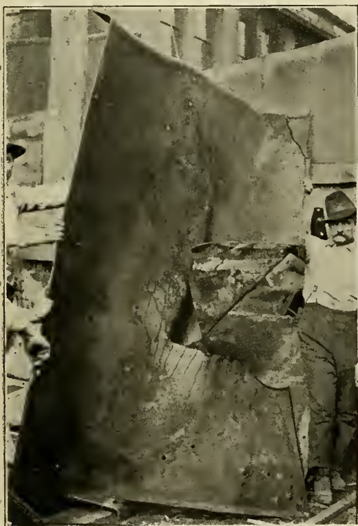
FIG. 28.—A TORN AND BENT SIDE SHEET AWAITING REPAIRS.
