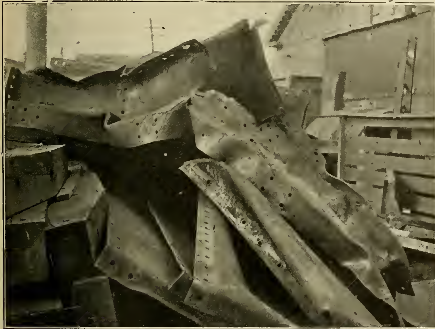
FIG. 32.—BENT AND TORN END SILL.
