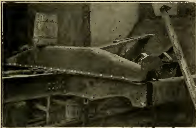
FIG. 39.—HOPPER CAR SIDE SILL BROKEN AT THE BOLSTER.
