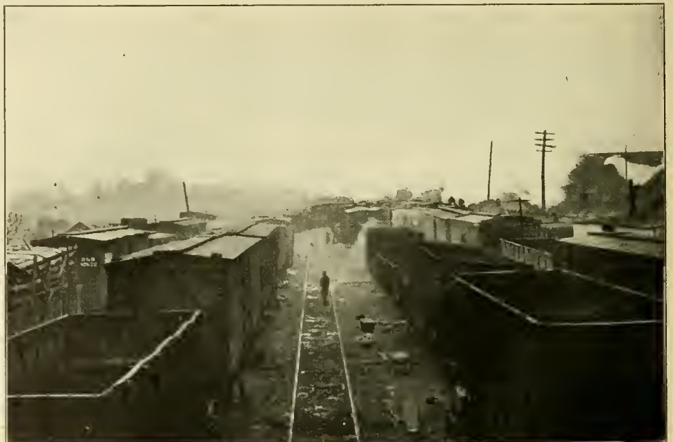
FIG. 11.—VIEW OF THE REPAIR YARD LOOKING WEST, FROM NEAR THE CENTER.
