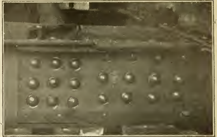
FIG. 38.—CENTER SILLS ON HOPPER CAR SPLICED IN FRONT OF THE BOLSTER AND AT THE REAR DRAFT LUG.
