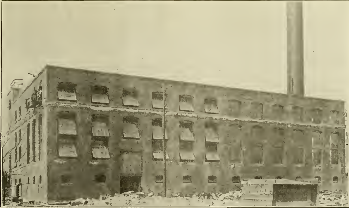
POWER HOUSE, HORNELL SHOPS—ERIE RAILROAD.
