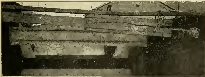
FIG. 12.—"BOX JACK" FORCING THE SIDES OF A CAR OUTWARD.
