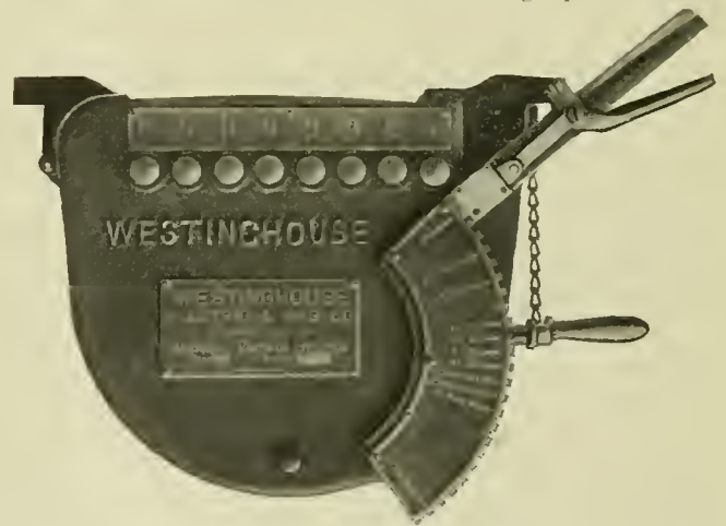
TOP VIEW OF MASTER CONTROLLER.
