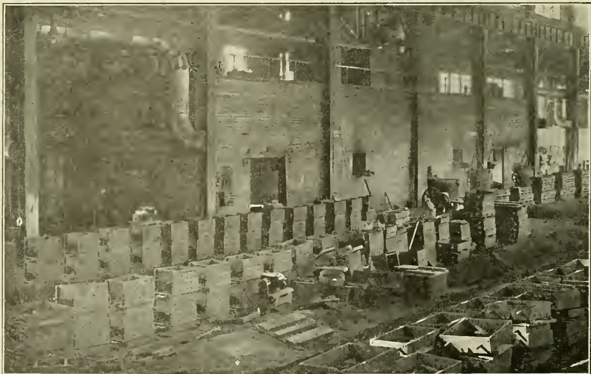
INTERIOR OF GREY IRON FOUNDRY—SOUTH LOUISVILLE.
