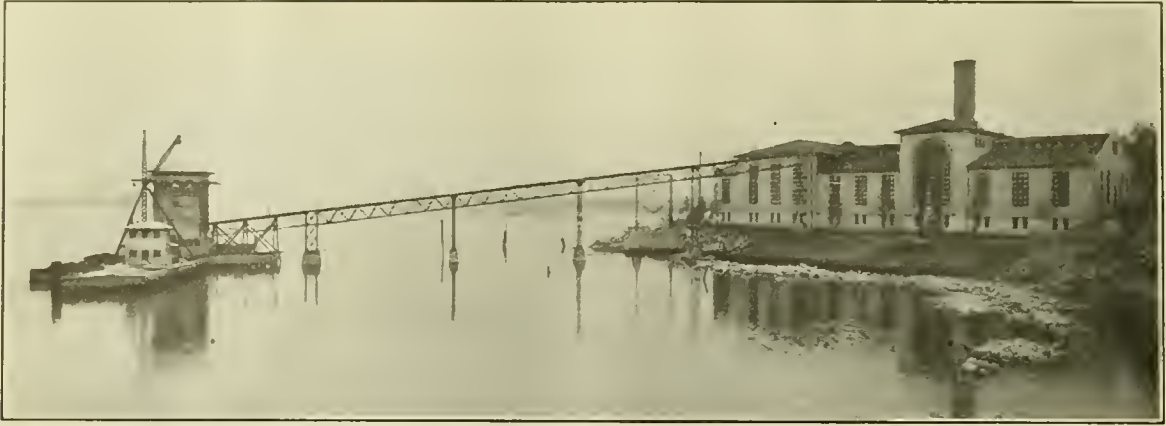
VIEW OF COS COB POWER HOUSE SHOWING COAL DOCK AND CONVEYOR.
