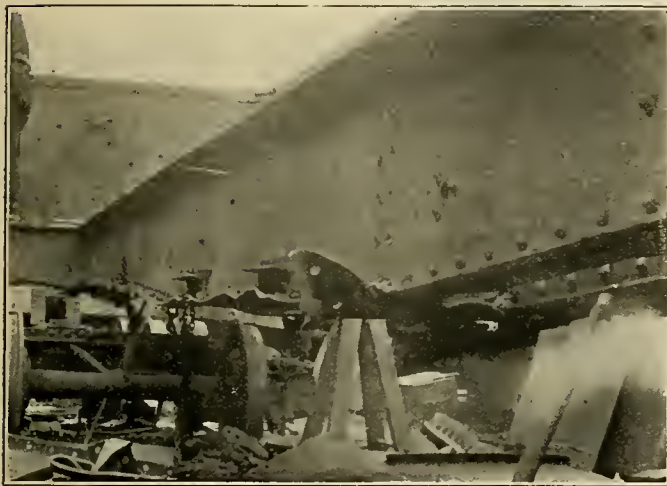
FIG. 49.—LOWER EDGE OF CENTER SILL DAMAGED ON CLASS O-17 GONDOLA CAR.
