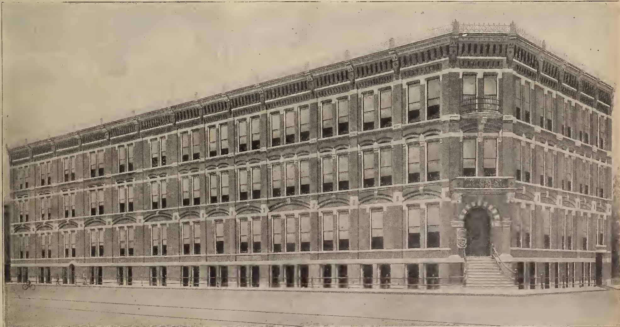
This Building is Owned and Occupied Exclusively by the Publishers of Farm and Fireside. It is Built of Red Pressed Brick, with White Stone Trimmings, 200 BY 75 FEET. To Accommodate the Growing Business a Large Addition was Built During the Past Year
