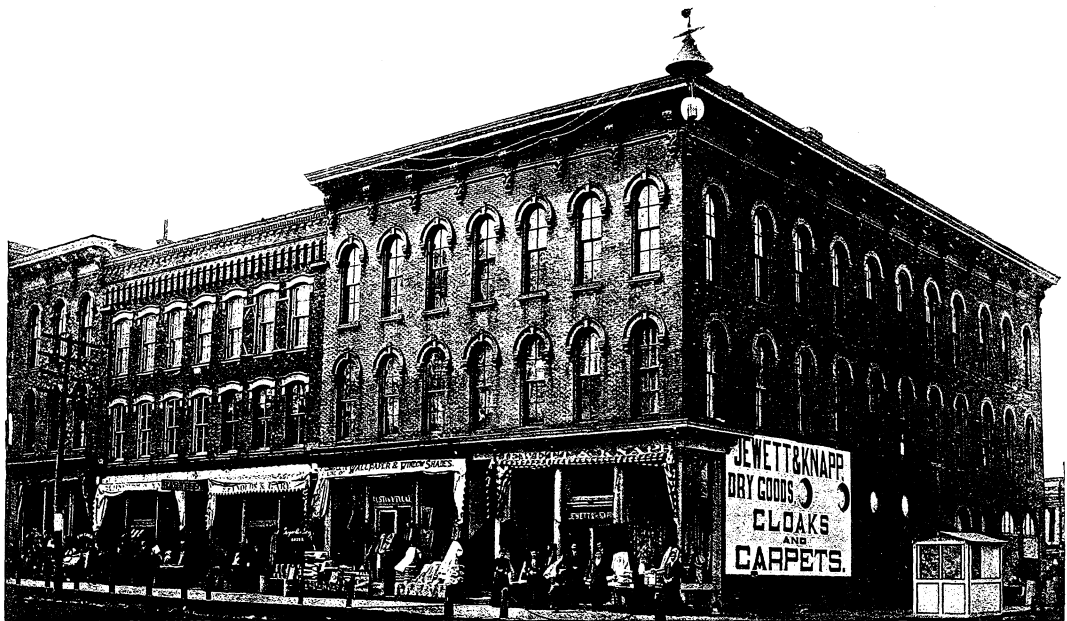
WEST SIDE SUPERIOR STREET—LOOKING SOUTH FROM CENTER STREET.
