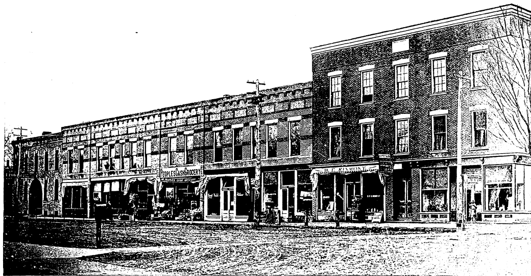
WEST SIDE SUPERIOR STREET--LOOKING SOUTH FROM ERIE STREET.
