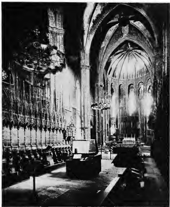
NAVE OF BARCELONA CATHEDRAL.
