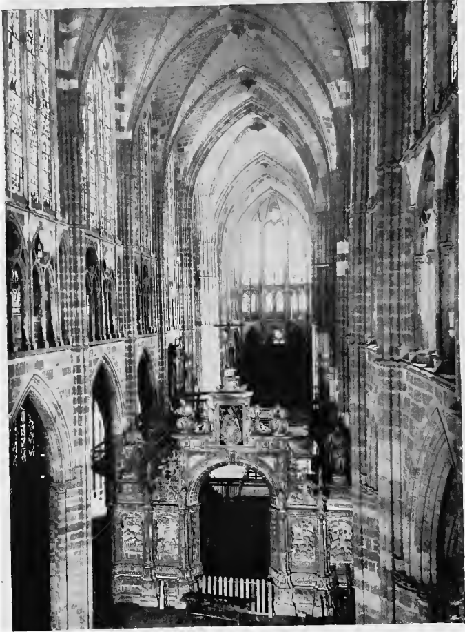
NAVE OF LEON CATHEDRAL.
