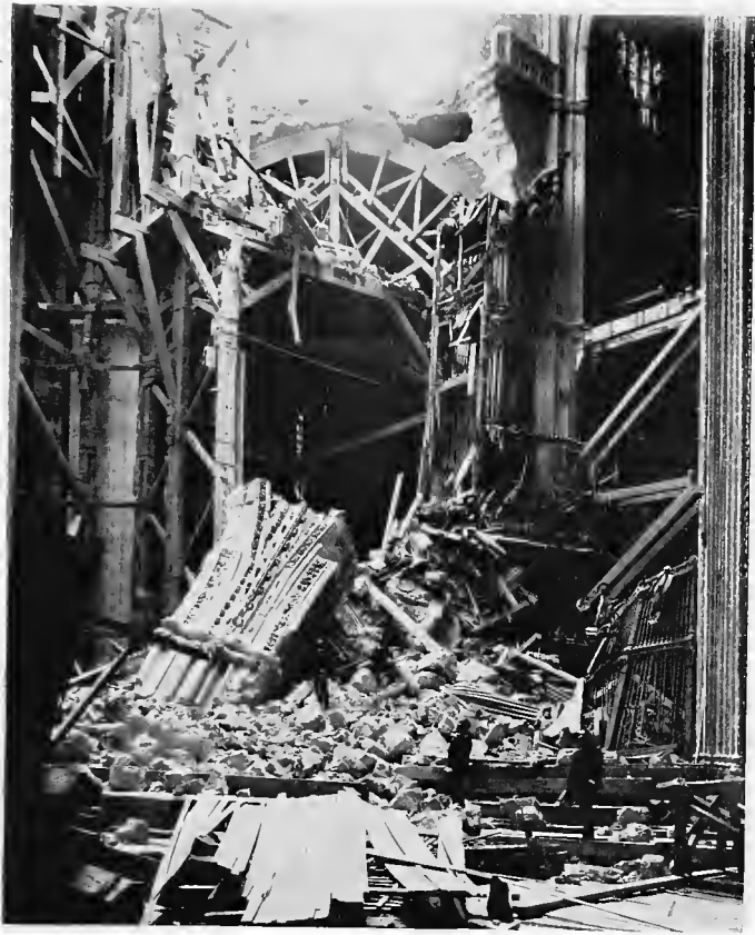
COLLAPSE OF THE CENTRAL VAULTS, SEVILLE CATHEDRAL.
