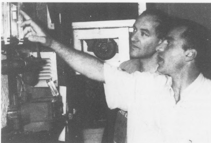
Mr. Musai, right, examines the chancery's air conditioning system.
