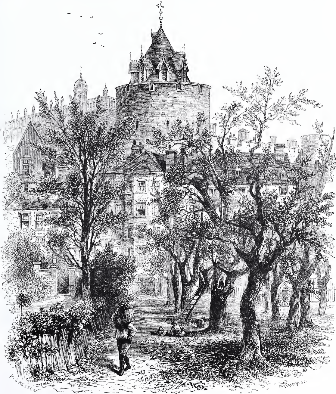
The Curfew Tower, Windsor.
