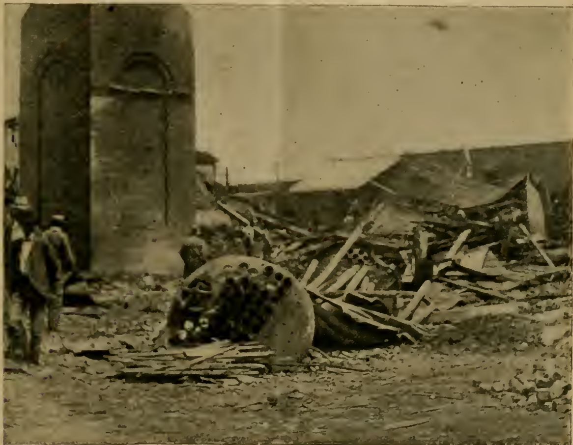
FIG. 3. — SHOWING THE EXPLODED BOILER.
