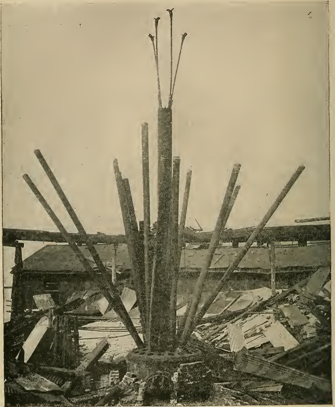
FIG. 2.— SHOWING THE EXPLODED BOILER IN DETAIL.
