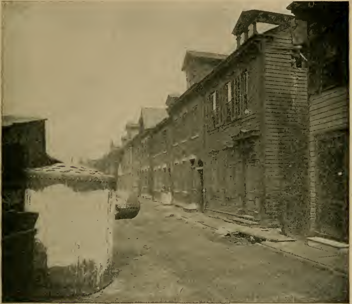
FIG. 3.—SHOWING WHERE THE UPPER DRUM FELL.
