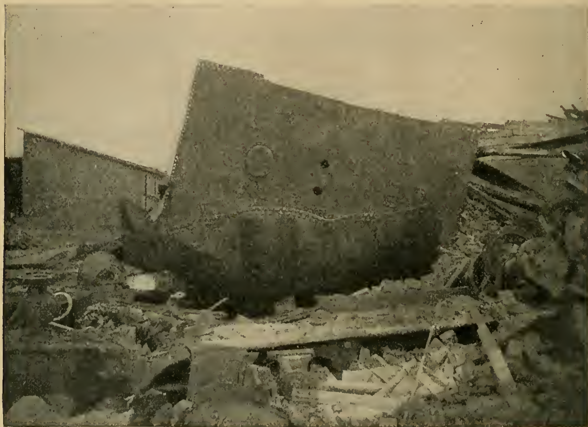
FIG. 2.—SHOWING THE SHELL OF THE BURSTED BOILER.
