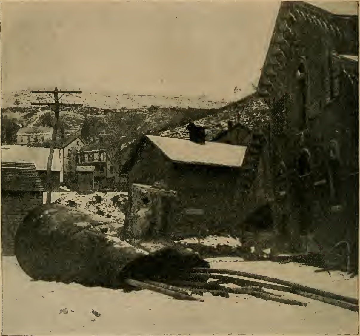
FIG. 2. — FORWARD PART OF THE BOILER, AFTER THE EXPLOSION.
