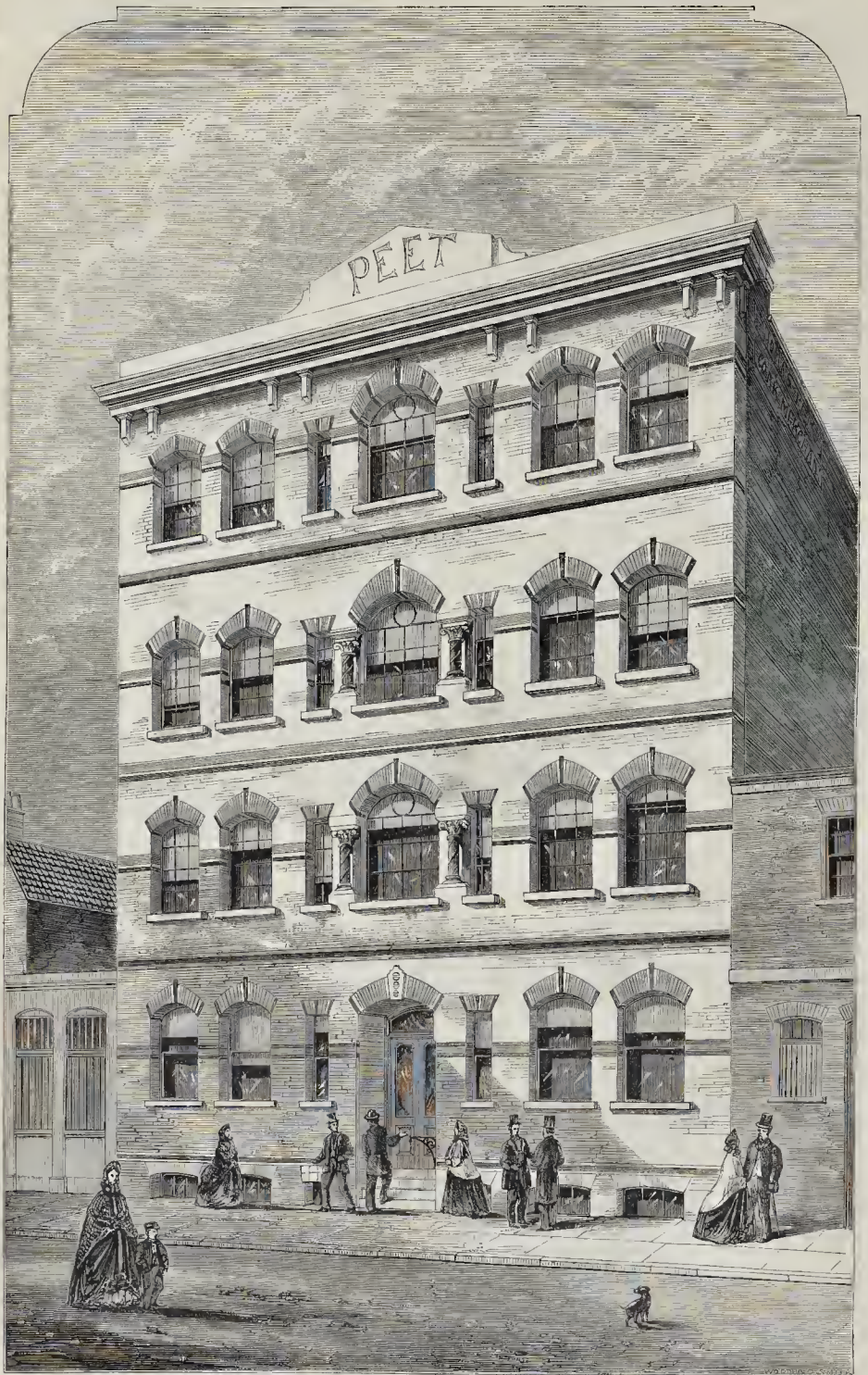
CORK WAREHOUSE, LANT STREET, SOUTHWARK.—MR. JOSEPH S. MOYE, ARCHITECT.
