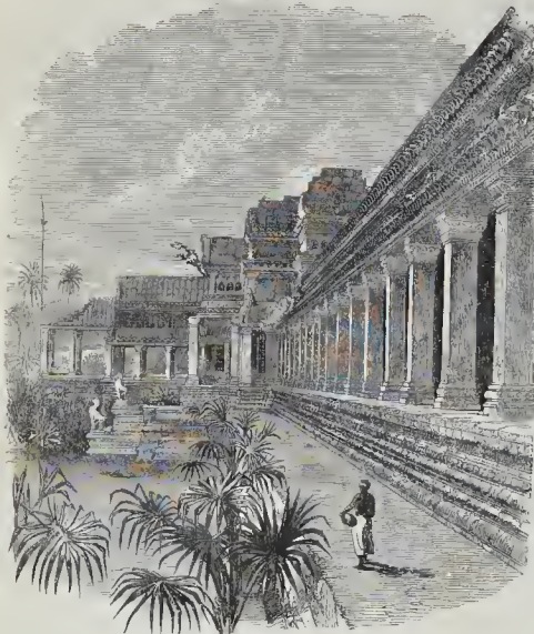
View of Exterior of Corridor.
