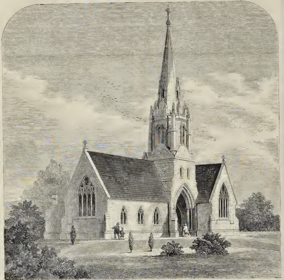
MARCH NEW CEMETERY, ISLE OF ELY, CAMBRIDGE. —Mr. G. W. STEPHENSON, ARCHITECT.
