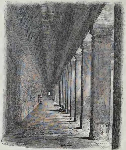
View of Interior of Corridor.
