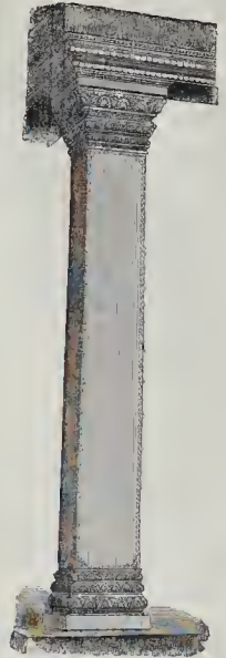
Pillar of Porch.
