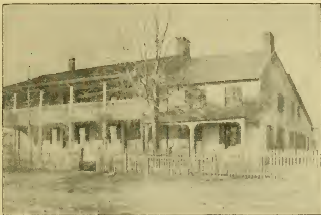
FOUR-MILE HOUSE, OPPOSITE CAMP CHASE.
