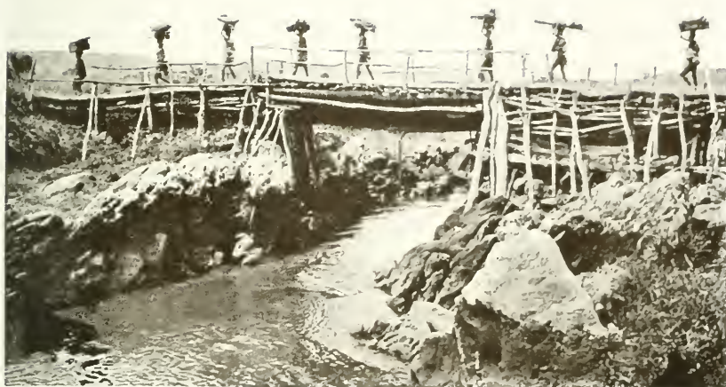
A BRIDGE ON THE HIGHWAY
