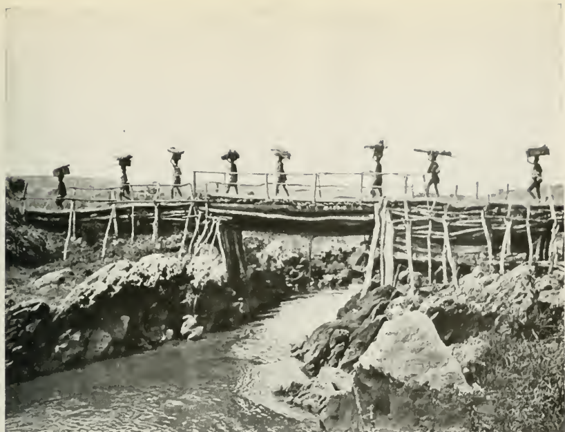
A BRIDGE ON THE HIGHWAY
