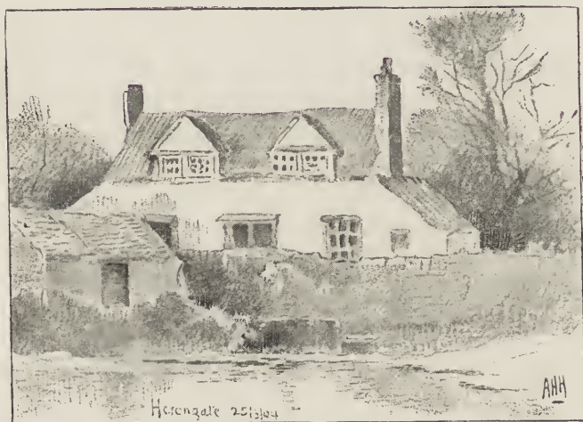
COTTAGE AT HERONGATE.
