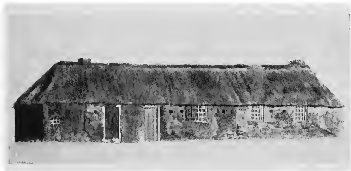
GUARD HOUSE, } GRAHAMSTOWN
