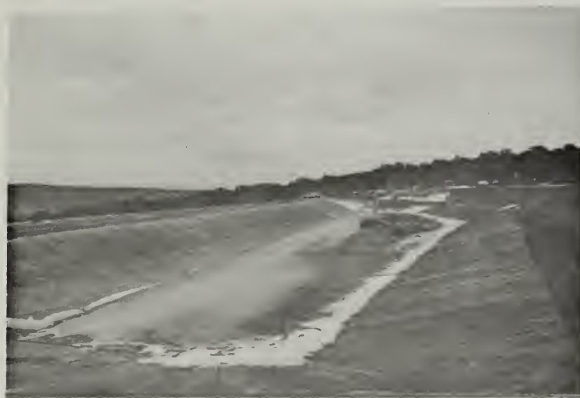
FIGURE 3-2-17 RETORT SOUR WATER POND CONSTRUCTION
