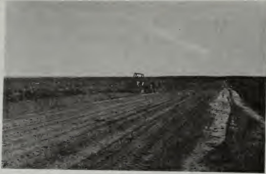
FIGURE 5-1-3 RECLAMATION OF AIRSTRIP BERMS
