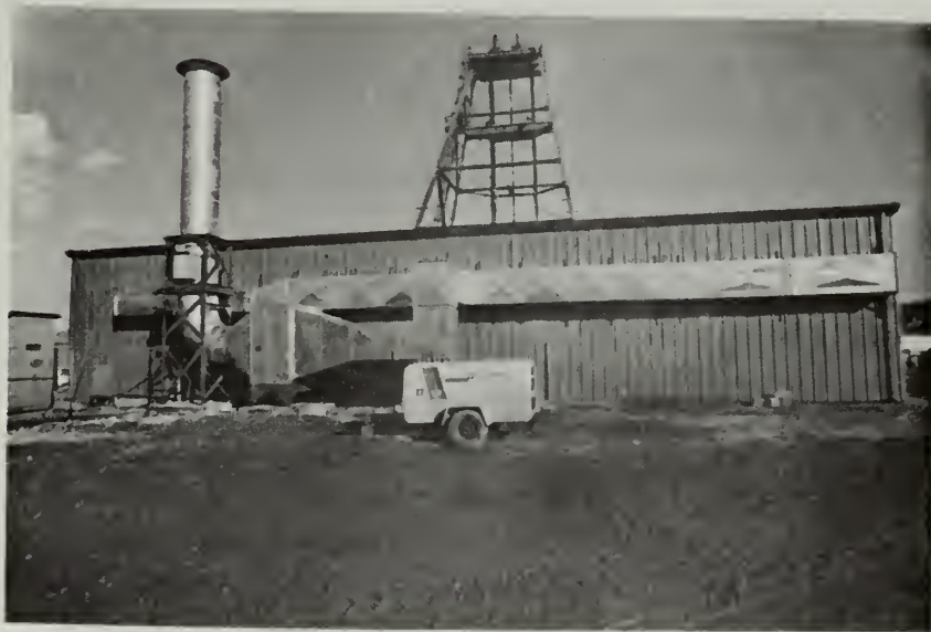
FIGURE 2-3-3 HOIST HOUSE VENTILATION AND FILTER DUCT
