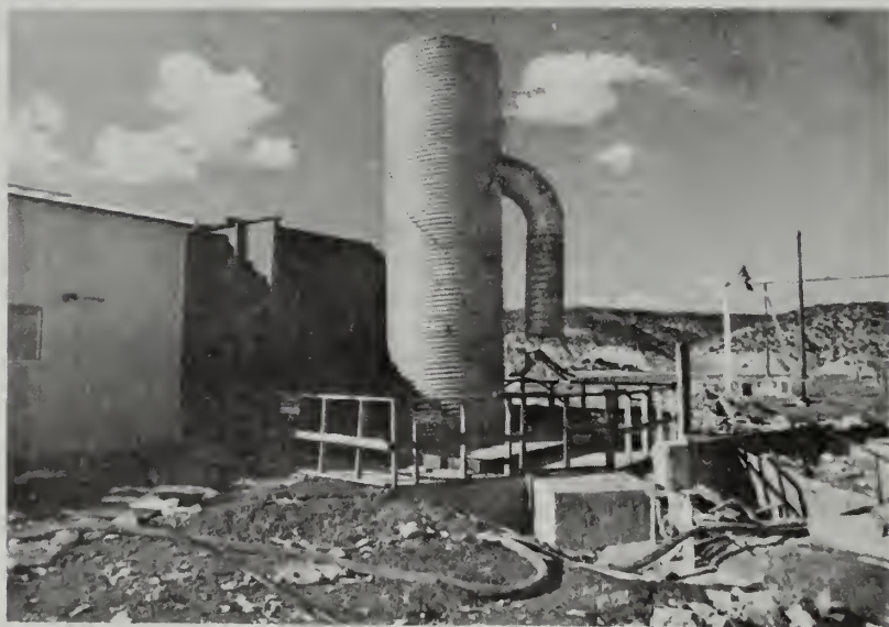
FIGURE 2-3-6 VENTILATION SHAFT COLLAR PRIOR TO INSTALLATION OF JEFFREY FAN
