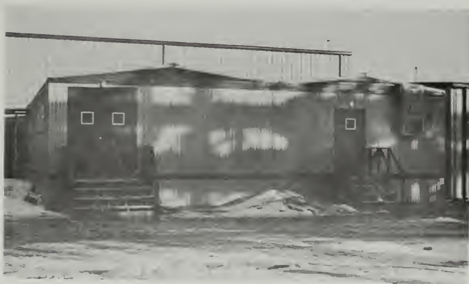
FIGURE 5-6-4 CONTROL ROOM BUILDING
