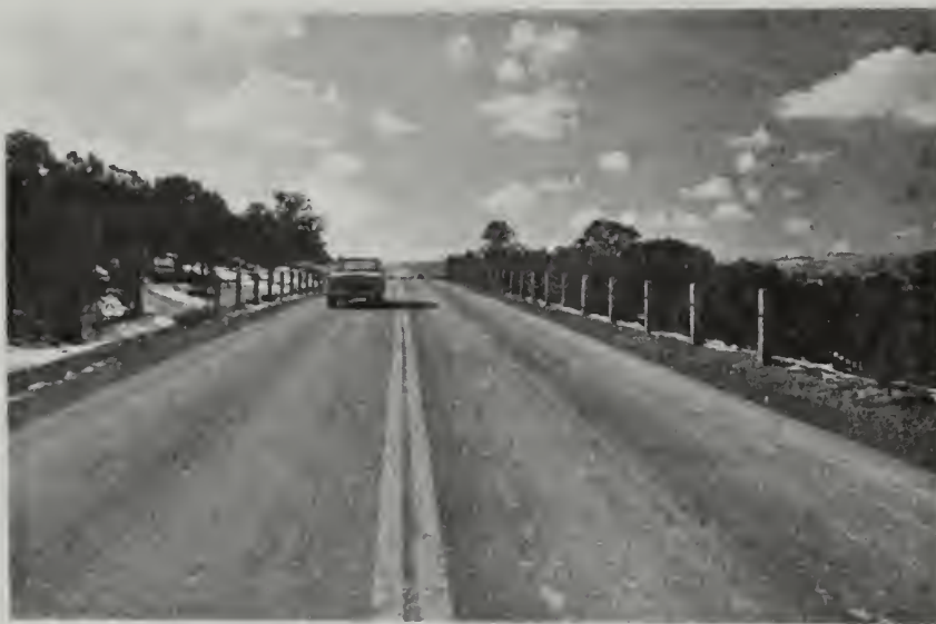
FIGURE 5-1-1 TRACT C-a PAVED ACCESS ROAD
