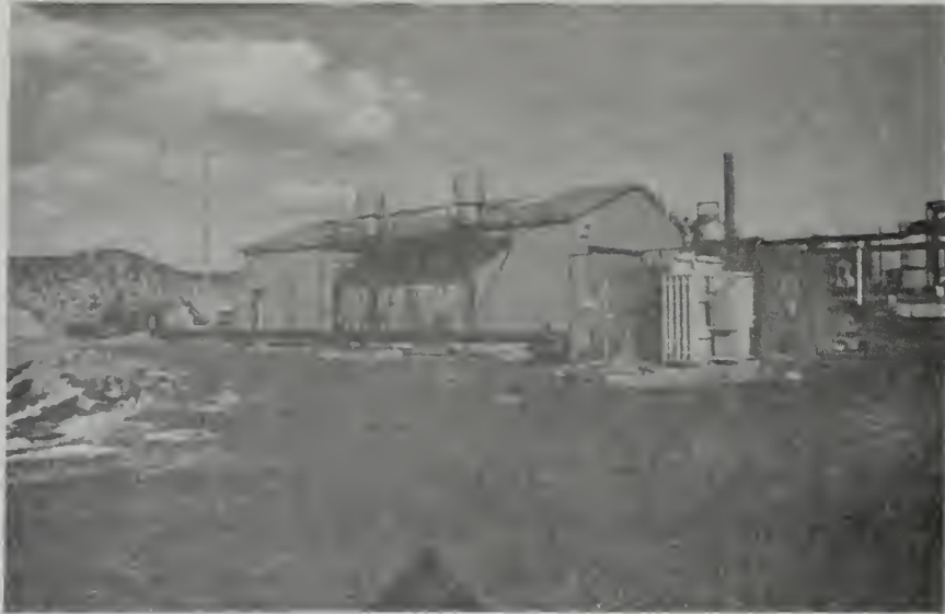
FIGURE 5-6-1 MINE COMPRESSOR BUILDING
