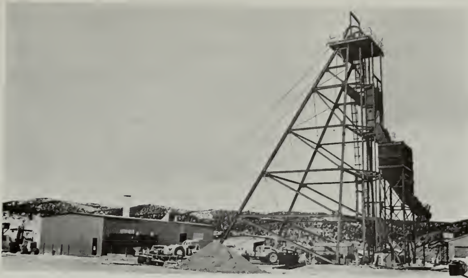
FIGURE 2-3-2 50 TON ORE BIN MOUNTED ON HEADFRAME
