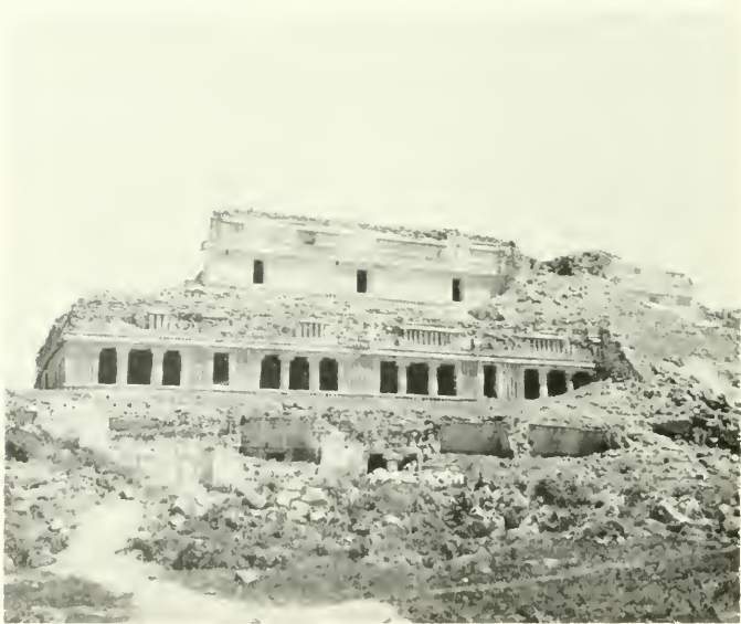
2. A palace-type structure of the Mayan ceremonial center of Sayil, Yucatan, Mexico. This handsome building, now largely in ruins, was built of rubble faced with cut limestone blocks and mortar. It is estimated to have contained about 100 rooms. It was probably constructed, at least in its final phases, between A.D. 600 and 900.
