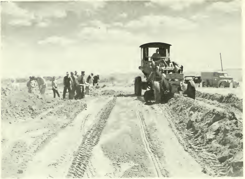
1. Using road-building equipment to clear overburden from village site.
