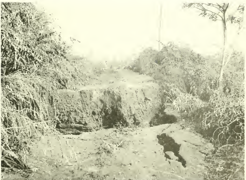
2. Four-foot fault scarp on north side of Kapoho graben, formed during the period of strong earthquake activity on January 13, 1960, immediately preceding the flank eruption.
