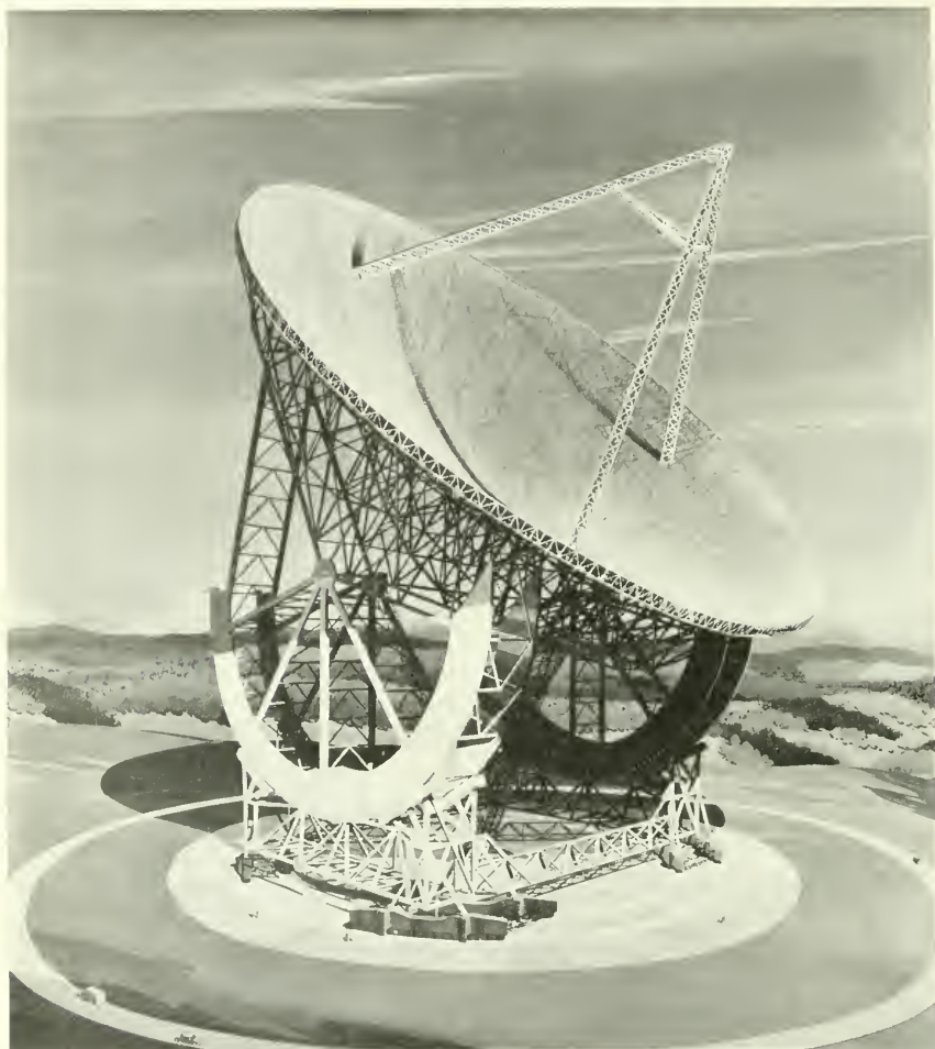
An artist's conception of the 600-foot antenna under construction for the U.S. Navy at Sugar Grove, West Virginia. This huge steerable paraboloid will be precise enough to work at wavelengths as short as the neutral hydrogen line at 21 centimeters. It will be an important tool for future planetary radar experiments. The installation, known as the Naval Radio Research Station, is to cost about $80,000,000. (U.S. Navy photograph.)
