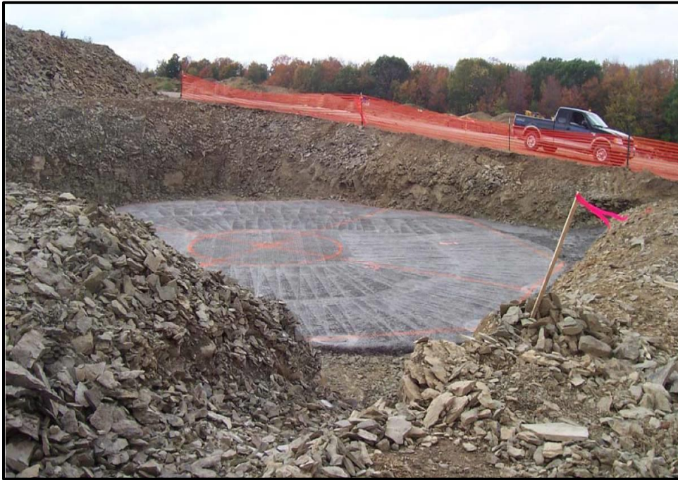
Figure 23. Excavated foundation area.
