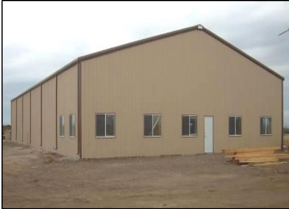
Figure 15. Typical O&M building.
