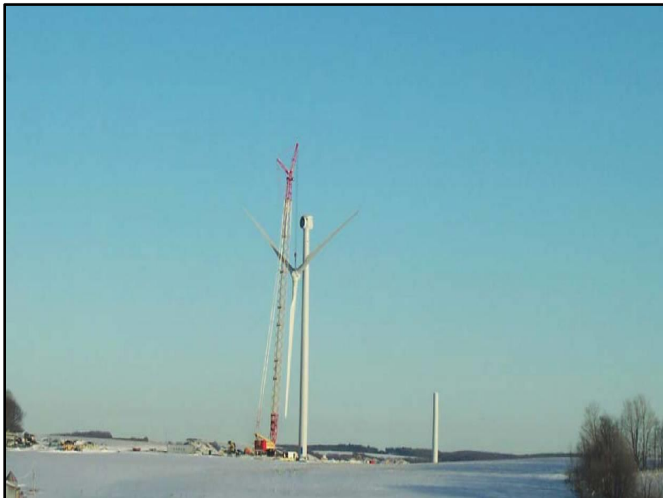
Figure 30. Installation of a rotor on a General Electric 1.5-MW wind turbine.
