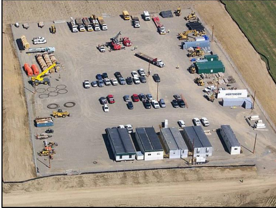
Figure 17. Typical storage/staging/laydown area during construction.
