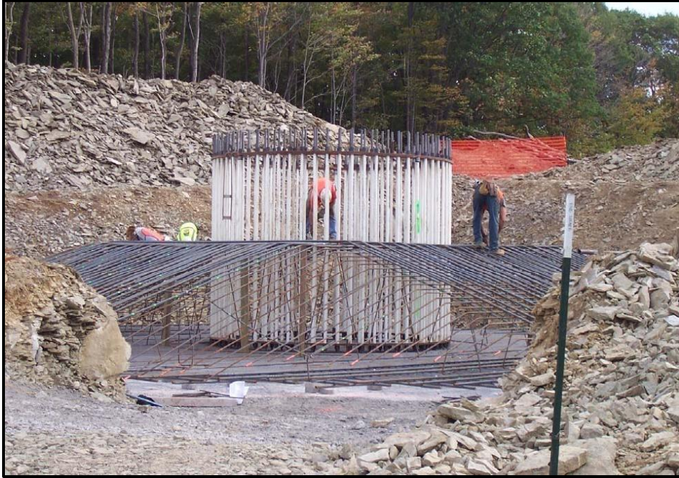
Figure 24. Foundation rebar and bolt cage.
