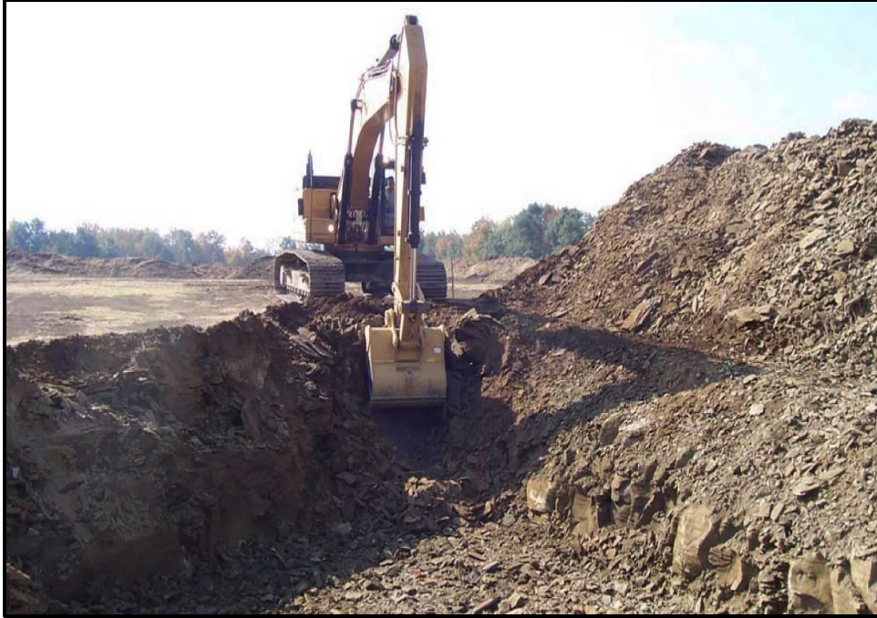
Figure 22. Excavating foundation hole.
