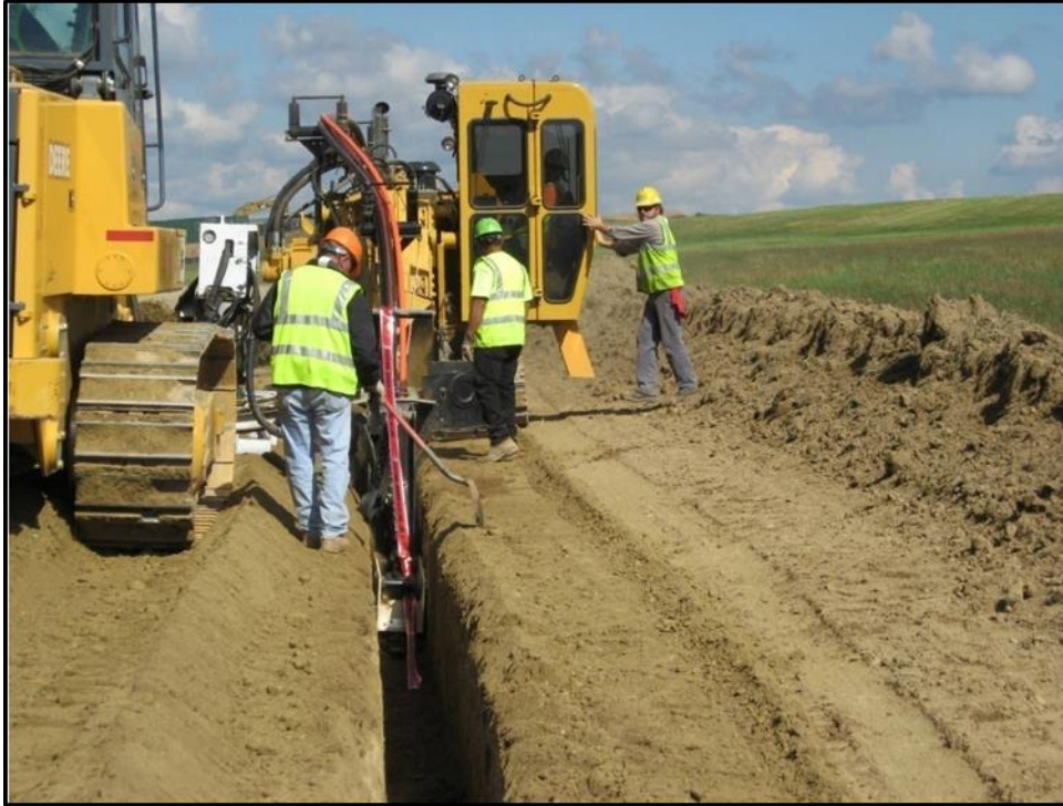
Figure 33. Typical underground collector cable trench.
