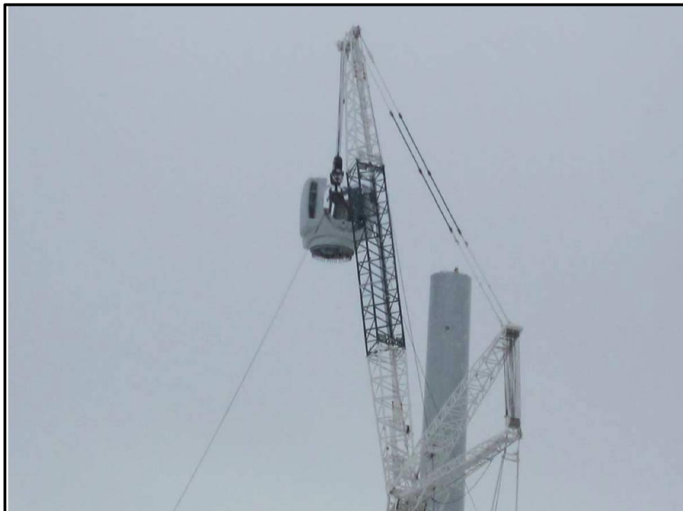
Figure 28. Wind turbine nacelle installation.
