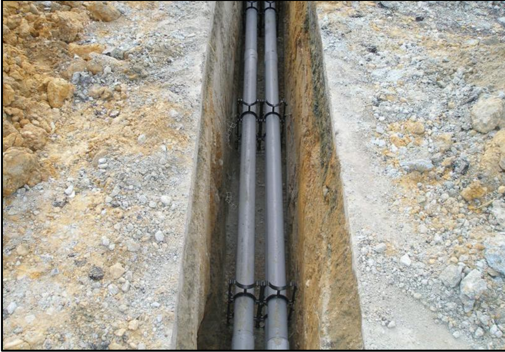
Figure 12. Typical collection lines.
