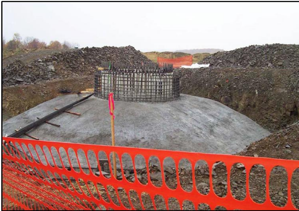
Figure 25. Typical spread-footing foundation.
