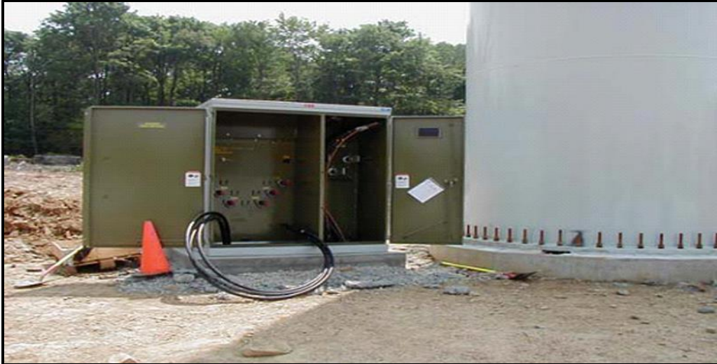
Figure 34. Typical pad-mounted transformer under construction.
