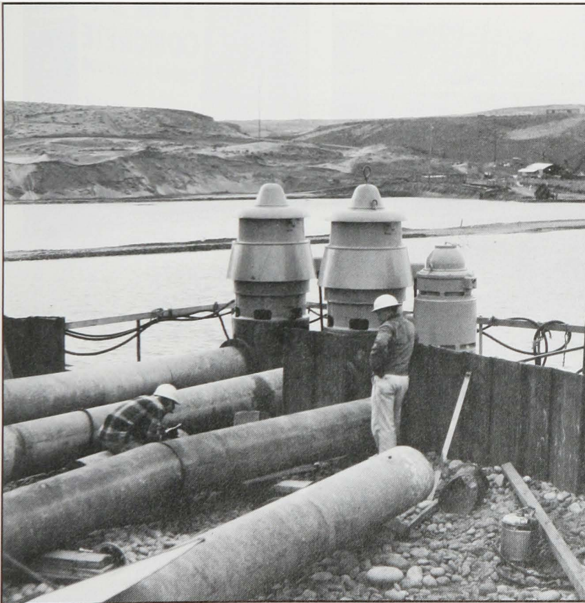
Installation of south shore cofferdam pumps used to keep work area dry during dam construction, December 1956.
