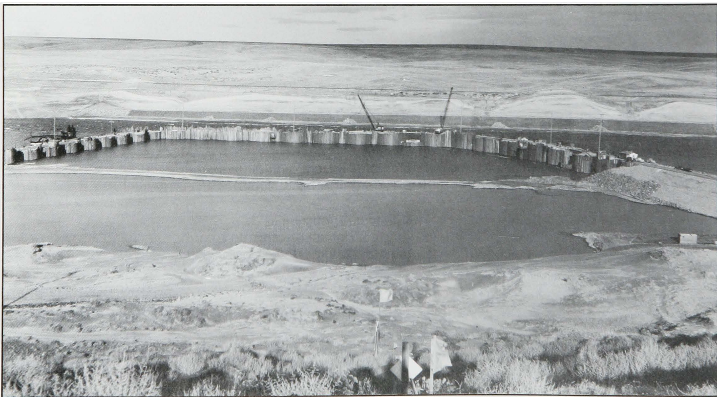
Completed south shore cofferdam for Ice Harbor construction, December 1956.
