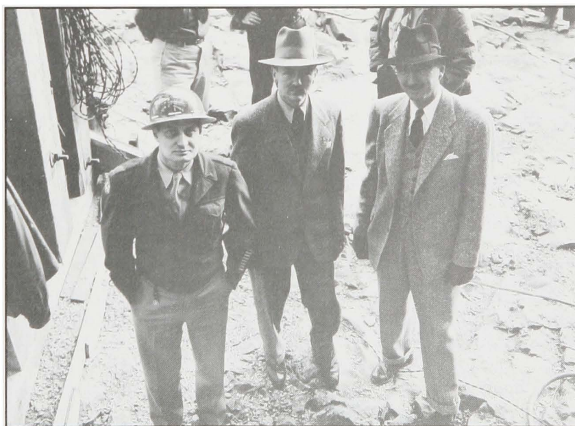
Col. William Whipple, center, first Walla Walla District Engineer, at McNary Dam construction site, 1948.
