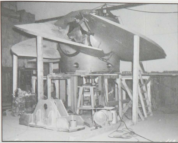
Turbine assembly awaiting installation in powerhouse, February 1960.
