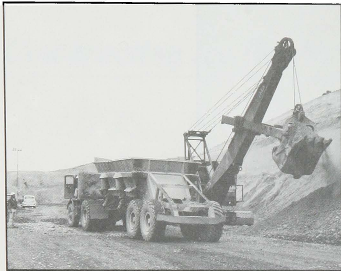
Excavation at Ice Harbor dam site, July 1956.
