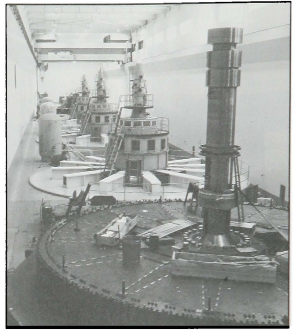
Lower Monumental second powerhouse construction, September 1978.
