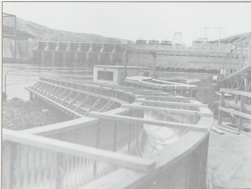
Construction of juvenile fish bypass system model at Lower Granite, March 1985
