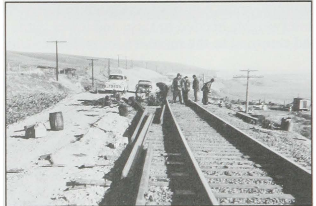
Relocation track for Spokane, Portland & Seattle Railroad.
