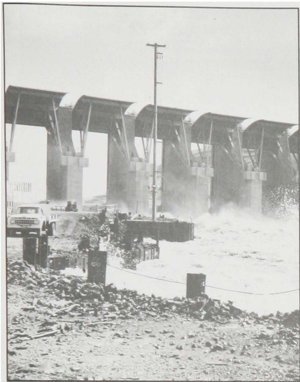
Construction at Lower Monumental Dam, 1960s.
