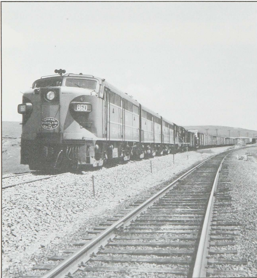
First freight train over the newly relocated tracks, 7 May 1958.
