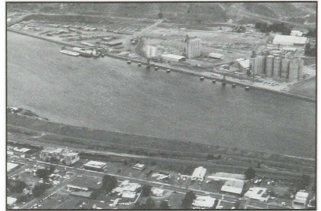
Eventually, the Walla Walla District constructed a levee system combining flood control and recreation as part of the Lower Granite project.
