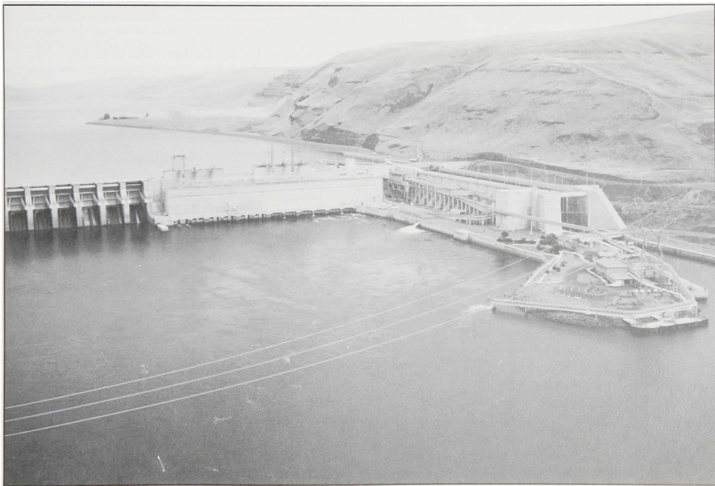
Little Goose Dam on the Snake River.
