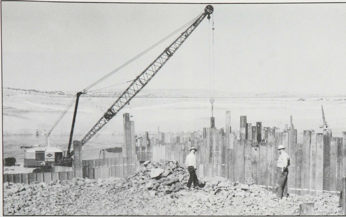
Placing stone topping in the cofferdam cells, September 1956.
