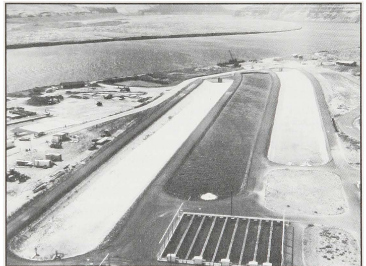
Lyons Ferry Fish Hatchery construction, 1983.
