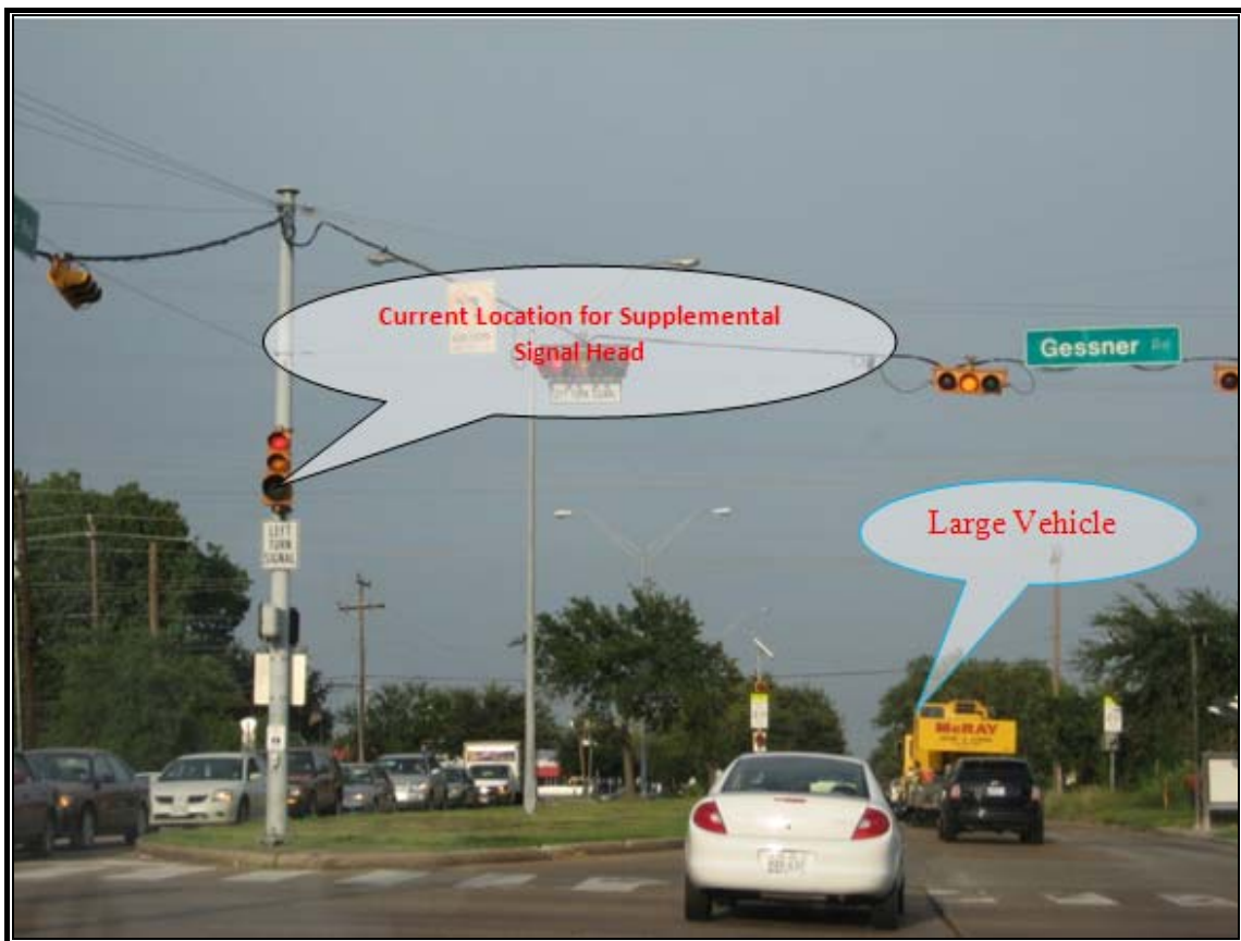
Figure 89: Current Supplemental Left-Turn Signal Head for the Intersection at Bellaire Boulevard and South Gessner Road in Houston, Texas
