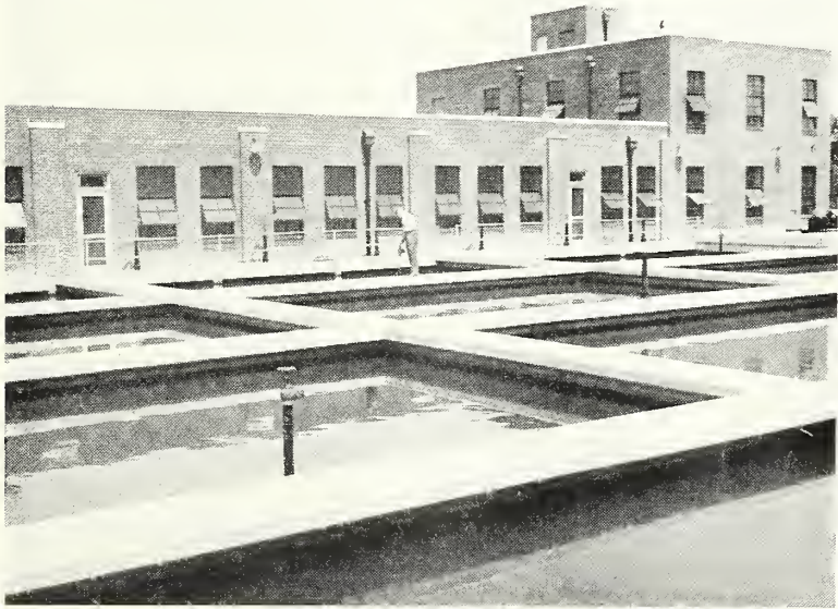
Concord's Modern Water Filtering Plant
