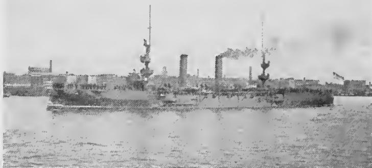
*New Orleans* (ex *Amazonas*), Protected Cruiser (British built). Dimensions, 330 x 44; draft, 17; displacement, 3,600. Speed, 20 knots. Main Battery, six six-inch, four 4.7-inch guns.
