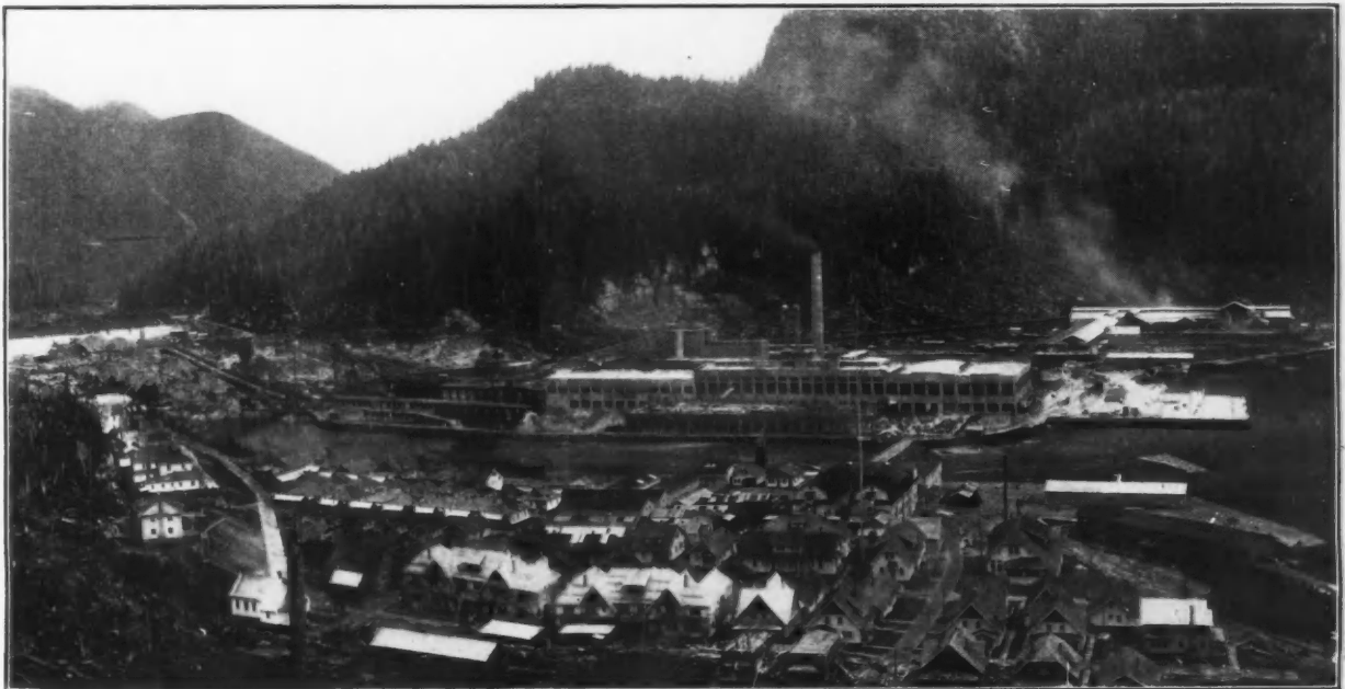
PLANT OF PACIFIC MILLS, LTD., RECENTLY COMPLETED AT OCEAN FALLS, B. C.
