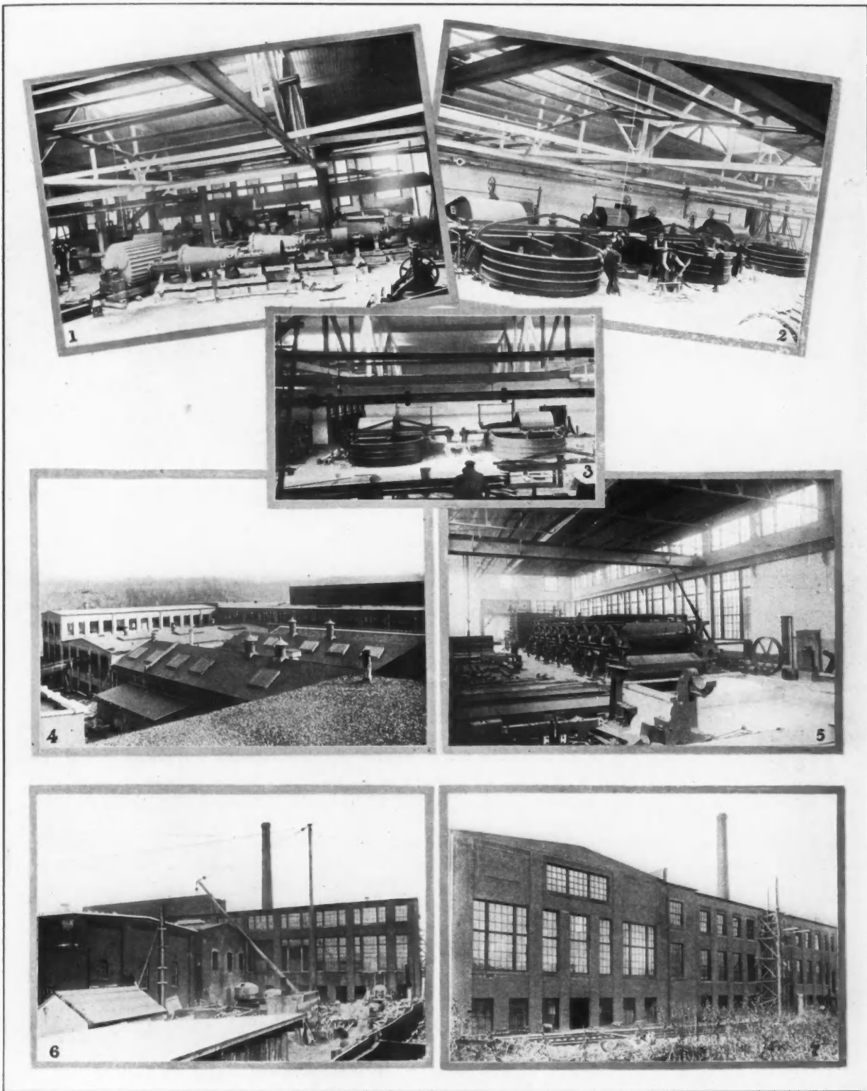
IMPROVEMENTS AT THE GILL DIVISION OF THE AMERICAN WRITING PAPER CO. No. 1. SHOWING 3 JORDANS IN PLACE IN NEW BEATER ROOM. No. 2. INTERIOR VIEW OF NEW BEATER ROOM. No. 3. INTERIOR VIEW OF BEATER ROOM. No. 4. VIEW OF MACHINE ROOM, BEATER ROOM, AND WASHER ROOM. No. 5. INTERIOR VIEW OF MACHINE ROOM SHOWING DRYER PART AND CALENDERS. No. 6. VIEW OF CONSTRUCTION YARD AND SOUTH WALL OF MACHINE ROOM. No. 7. WEST ELEVATION OF MACHINE AND WASHER ROOMS.
