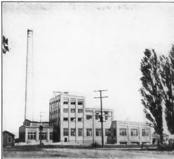
FRONT VIEW FILER FIBRE CO.
