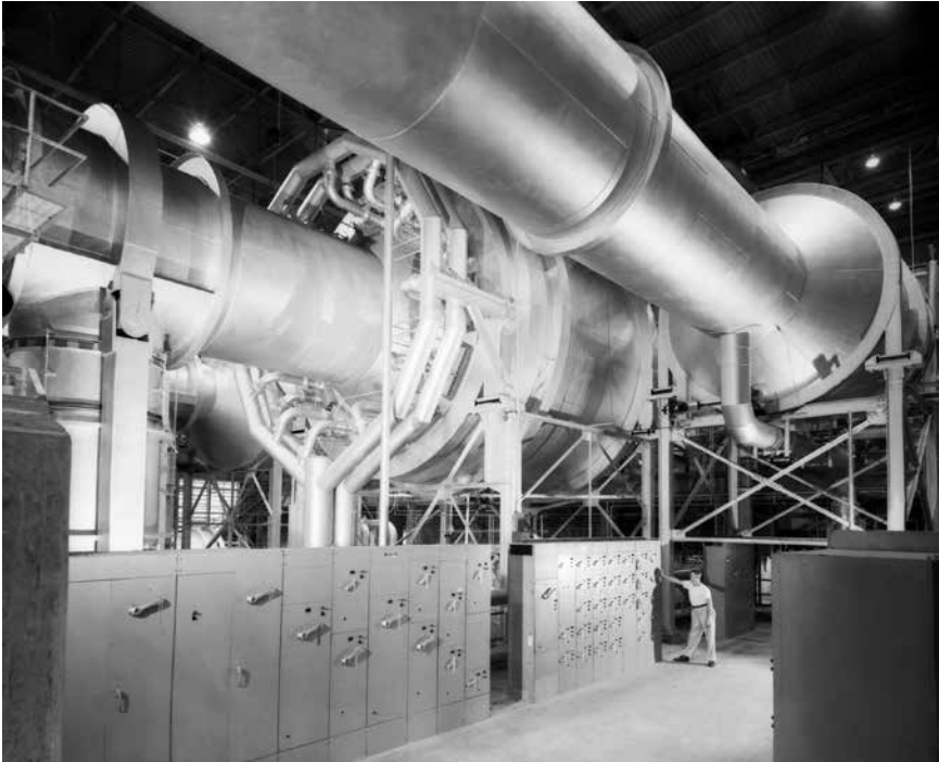
Langley's Unitary Plan Wind Tunnel, shown here upon completion in 1955, had two 4-by-4-by-7-foot test sections and could generate speeds up to Mach 4.63. (NASA)
