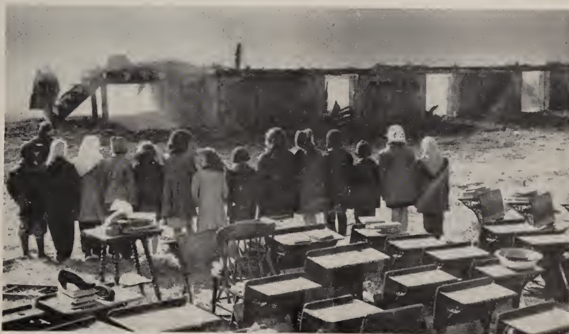
School building destroyed by fire in Bethel Township, Pa., but children were saved.
