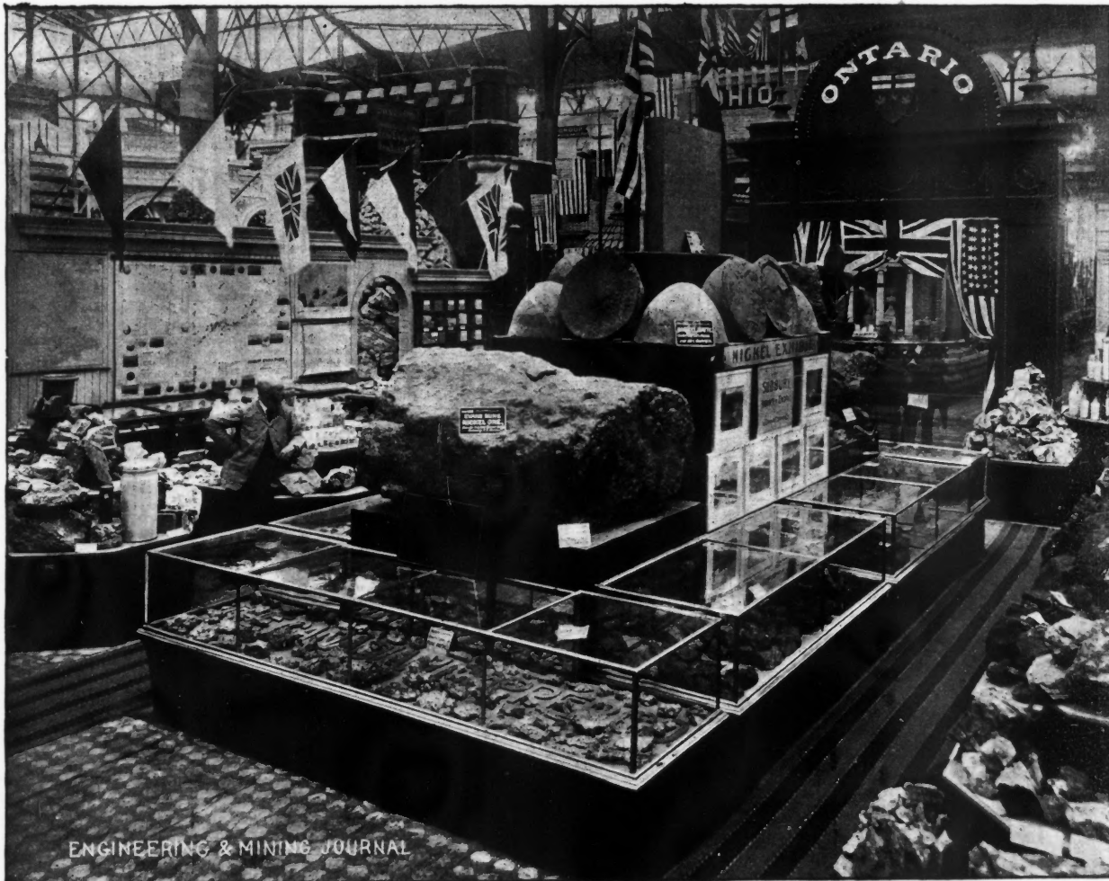
EXHIBIT OF THE CANADIAN COPPER COMPANY AT CHICAGO.
