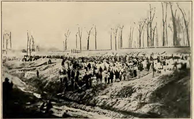
PRIMITIVE DRAINAGE AT CAMP MORTON
