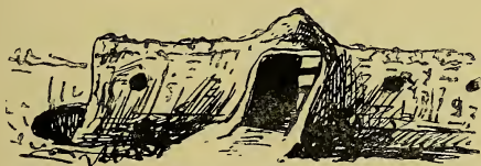
THE ENTRANCE GATE OF A VILLAGE IN KAVIRONDO.
