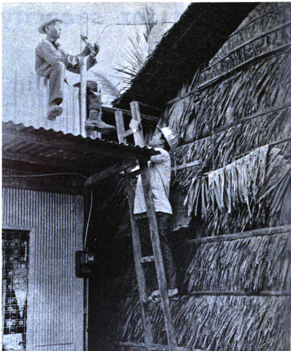
Members of rural electric co-ops provide their own internal wiring and fittings after house connections have been made by linesmen of co-ops.
