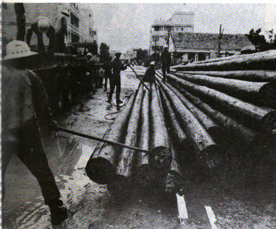
Poles arrive in An Giang from Phan Rang pole treatment plant to enable one of south Vietnam's three rural cooperatives to light up the hamlets.
