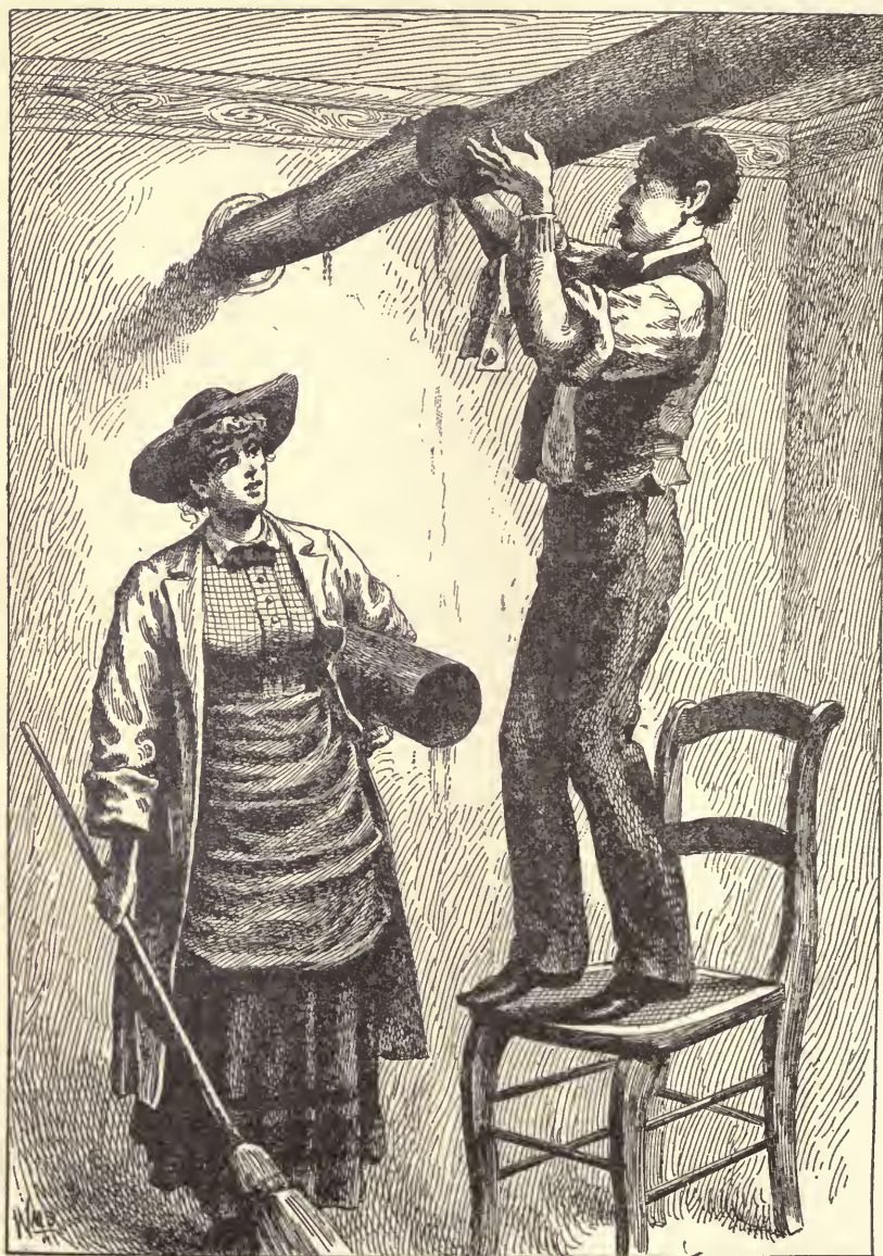
PUTTING UP A STOVE PIPE.
