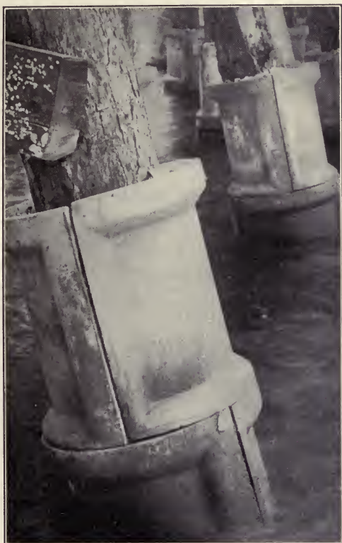
FIG. 61.—Piles protected by pipes and sand. 2
