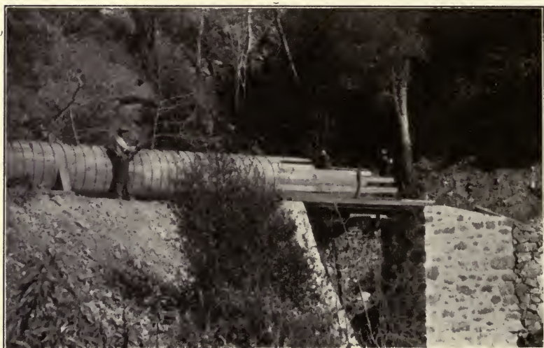
FIG. 29.—Assembling parts of redwood stave pipe.
