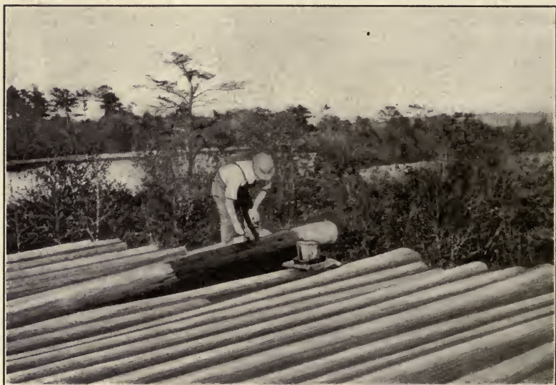
FIG. 75.—Treating poles by brush method. 1
