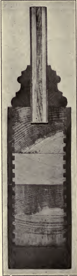
FIG. 84.—Section through door stile.
