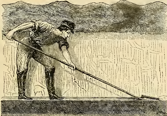
POSITION OF WORKMAN, AND USE OF FINISHING SCOOP.
