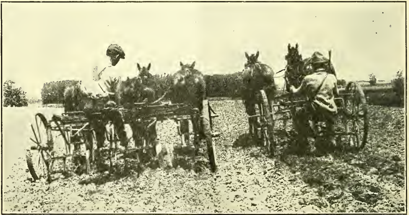
FIG. 8.—One man and three horses on a two-row cultivator accomplish nearly twice as much work as one man and two horses on a one-row machine.
