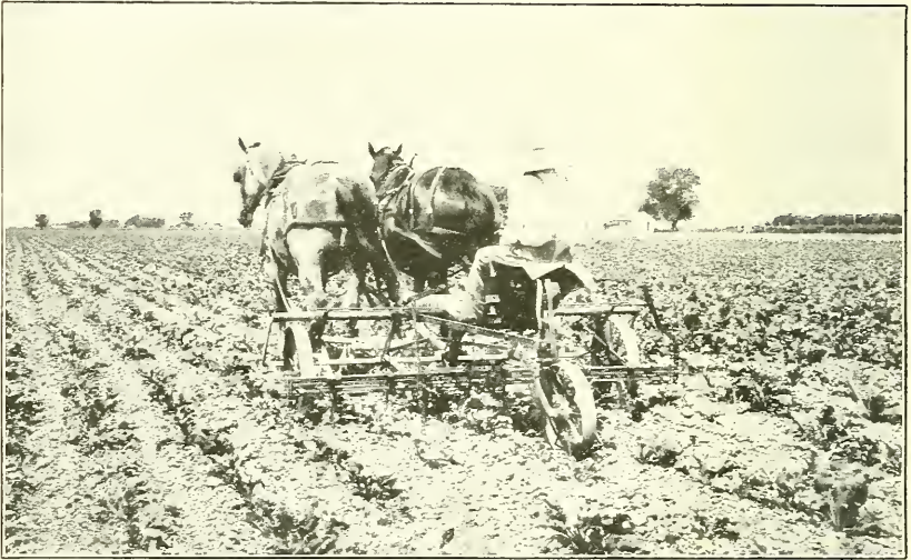
FIG. 1.—A 4-ROW CULTIVATOR, WHICH IF NOT CAREFULLY USED MAY DESTROY A GOOD STAND OF BEETS.
