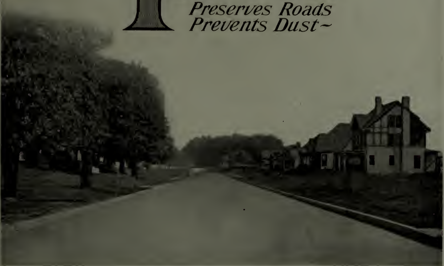
Cowden Avenue, Memphis, Tenn. Constructed with Tarvia X.
