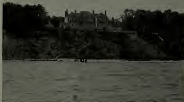
The Stonehill residence at Glencoe as seen from Lake Michigan. Along here the lake bluff reaches its greatest height and the ravines their greatest depth
