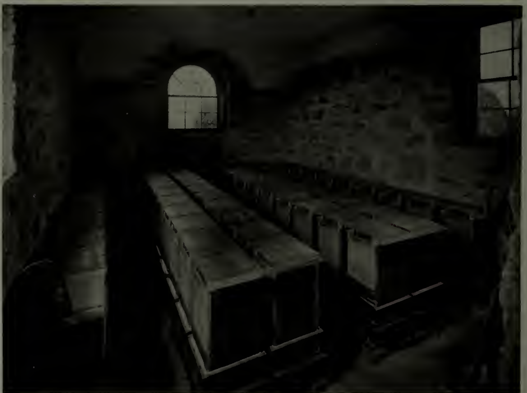
For a large plant, too, the capacity of the storage battery must be correspondingly greater, and a separate dry and well lighted room is usually provided for it
