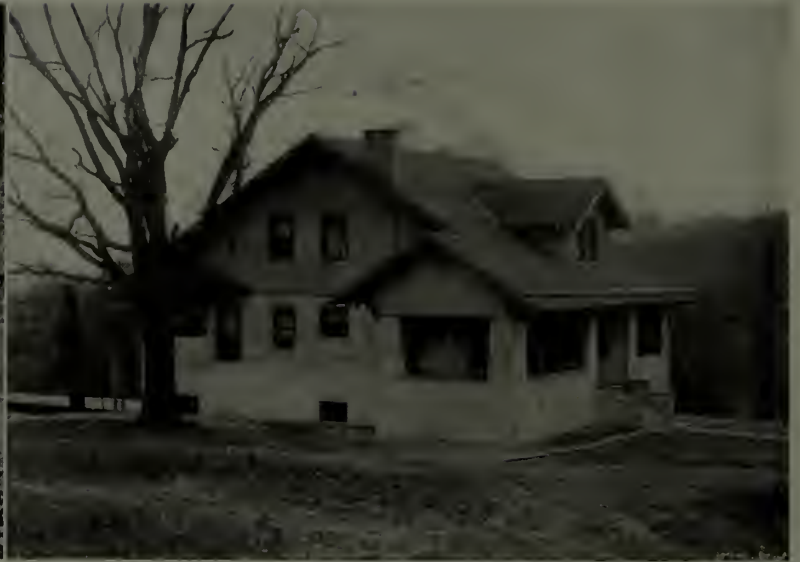
A stucco house with slate roof, the walls tinted in two tones
