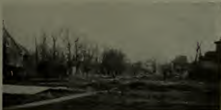
2. Six years ago, when the soil was first prepared for lawn and borders. Looking east from about the centre of the lot
