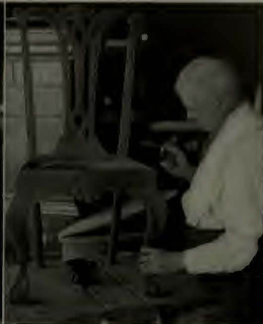
Each coat of shellac must be applied evenly and quickly and allowed to harden before being rubbed down
