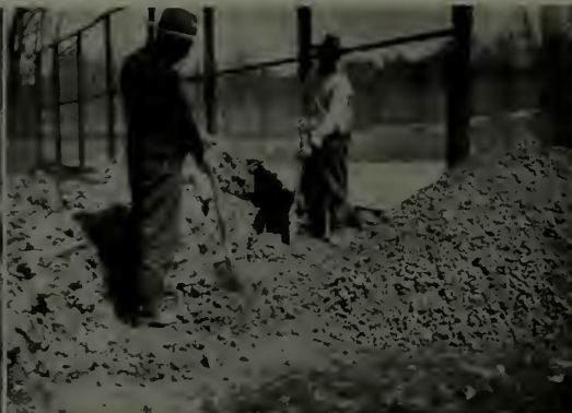
Chopping up the clay to facilitate its amalgamation and keying
