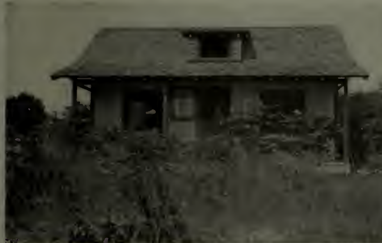
Front view of the $450 bungalow. Only by the elimination of a chimney and all mason work was such a price made possible
