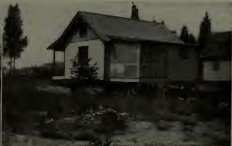
The 9-foot lean-to at the back of the house provides space for a compact little kitchen and a screened-in porch for summer dining
