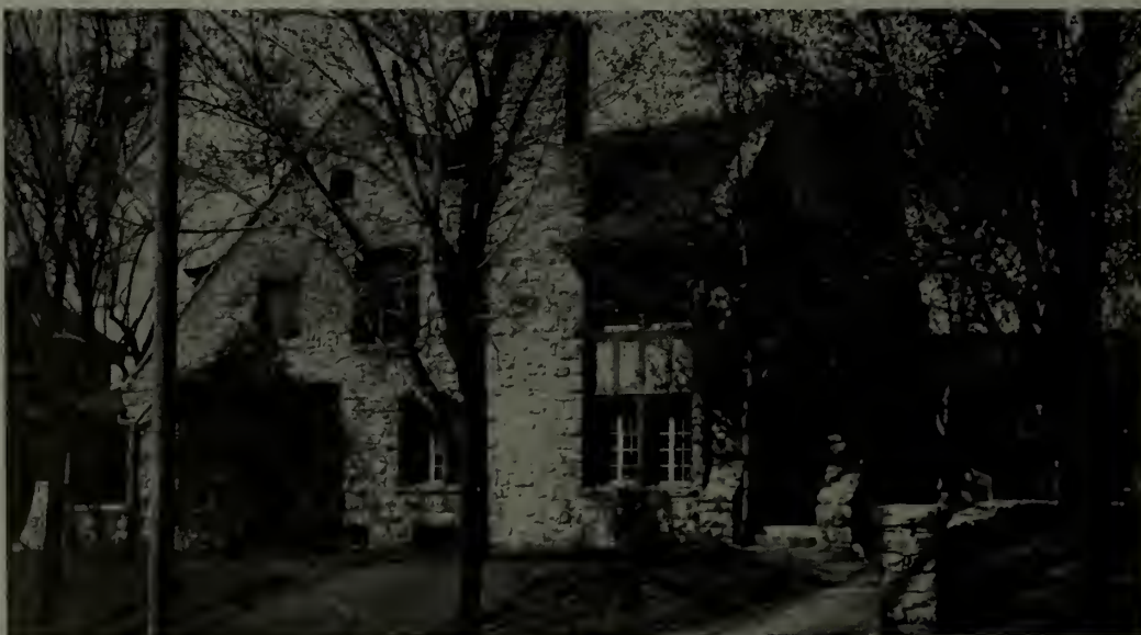
"Branches" is a native stone house, of simple but attractive exterior, built to the slope of the ground
