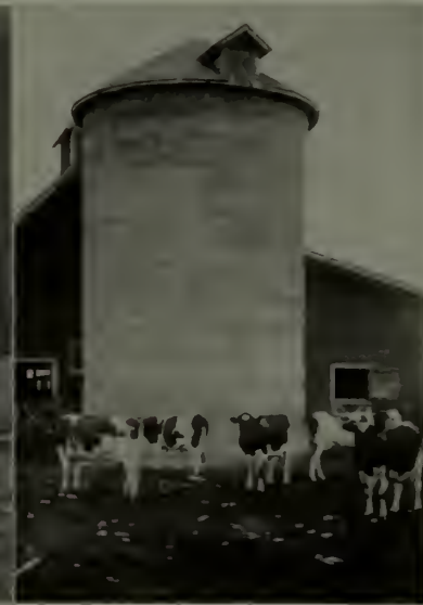
The size of the silo is determined by the number of cows kept
