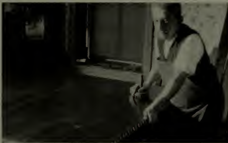
The wax is applied with a short-bristled brush. Rub slowly with the grain of the wood. In polishing, use slow, circular movements
