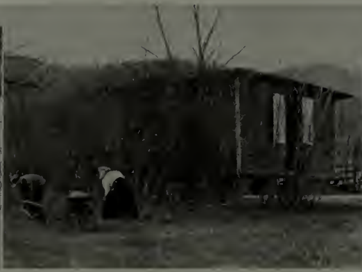
Breaking ground for a flower bed. The houseboat in position ready to be raised
