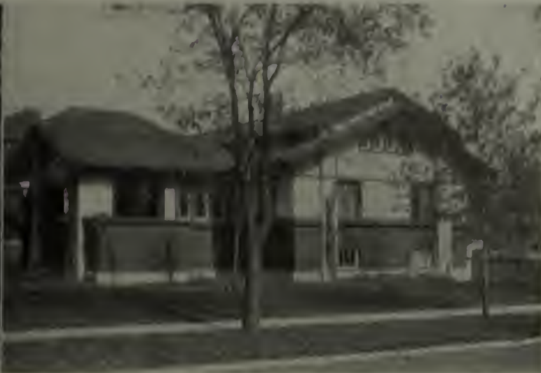
A bungalow near Chicago, showing many insurgent features. Tallmadge & Watson, architects
