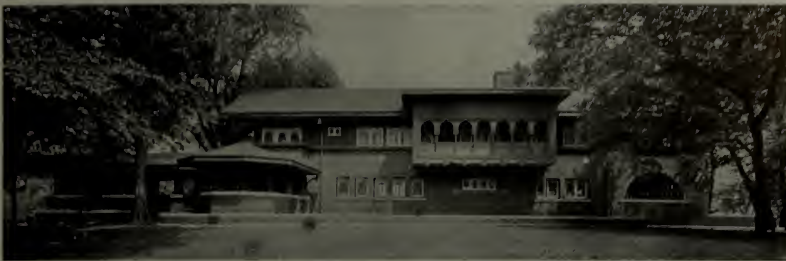
A typical example of the work of Louis Sullivan. The long horizontal lines, the use of the arch, the casement windows of unique design and their unconventional grouping, are all insurgent features
