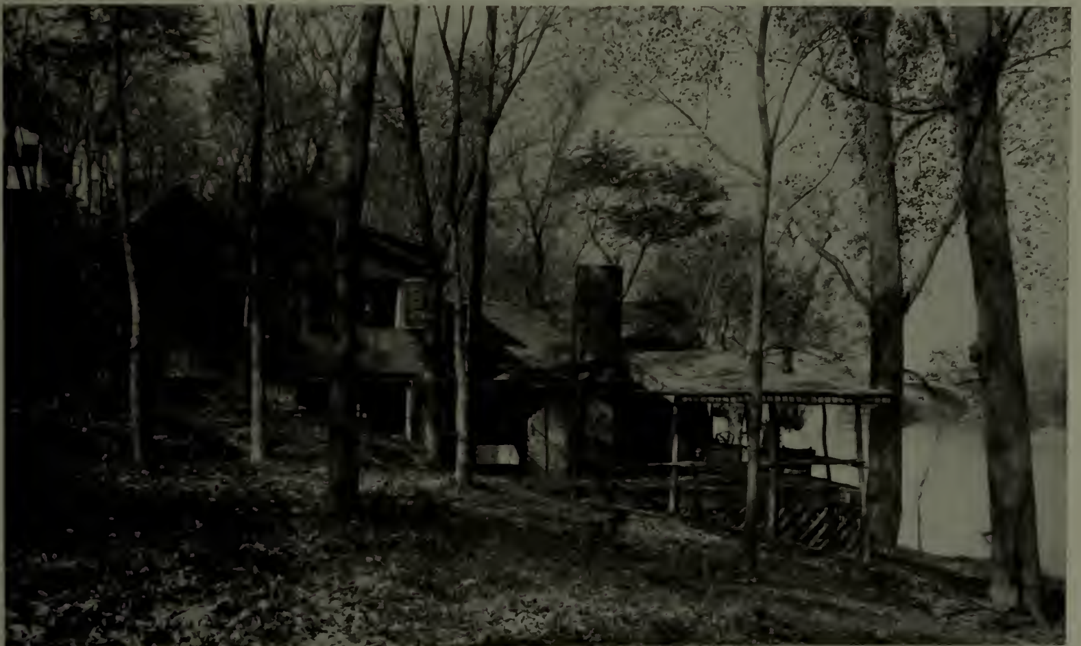
The bungalow that started life as a boat-house. It is built largely of saplings and logs, and cost only $1,500
