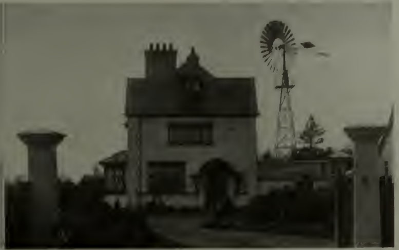
In England more than here windmills are used to generate electricity and charge storage batteries which ensure continuous current
