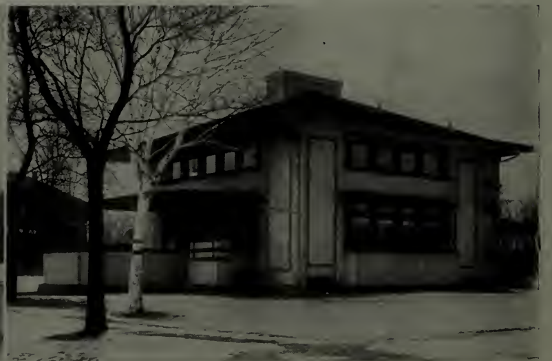
An inexpensive cement house by Wright, showing the pier and curtain-wall construction at its best. Note the treatment of the chimney, windows, and porch
