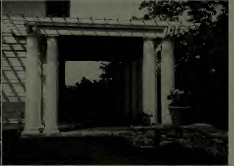
This pergola serves to unite the house with its site. Note the rough stone wall which separates the dressed ground from the wild
