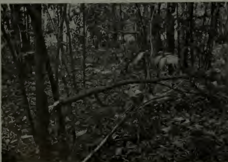
Blazing the way for the wood road. This was done by cutting small trees and bending them in the direction the road was to take
