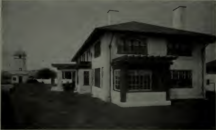
East view, showing the lawn and water tower. The exterior of the buildings and of the fence wall is cement; the sea wall, reinforced concrete, 14 feet high. The grounds comprise three quarters of an acre, with about 300 feet of shore front
