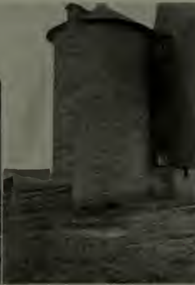
Concrete block construction is ideal for both appearance and durability
