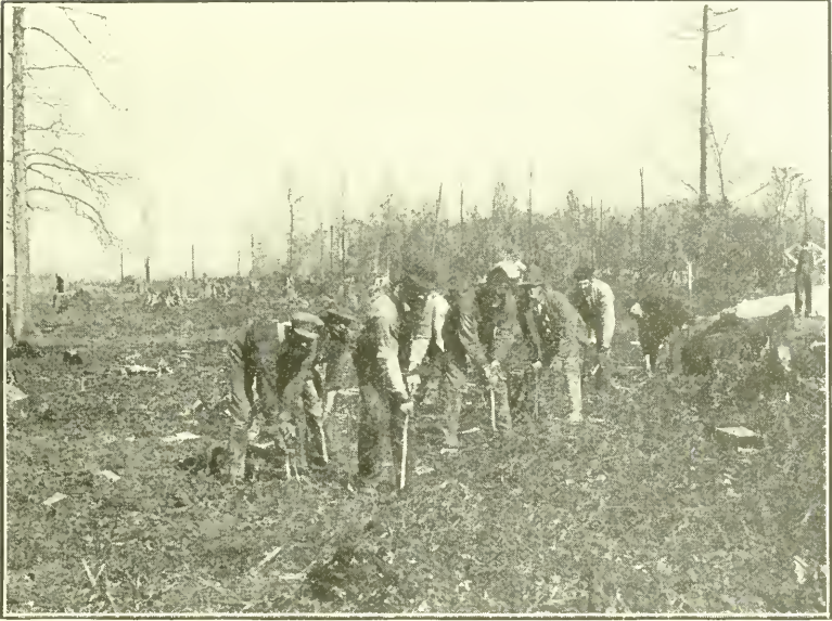
1. BORING THE HOLES FOR A DITCH
