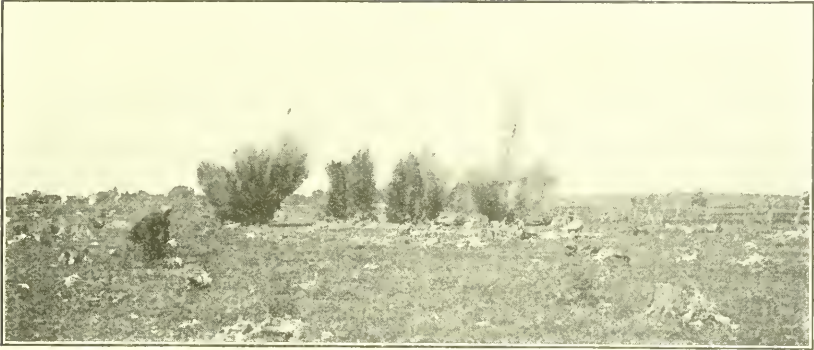
BLASTING STUMPS ELECTRICALLY
