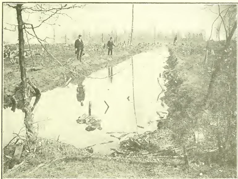
4. THE COMPLETED DITCH
